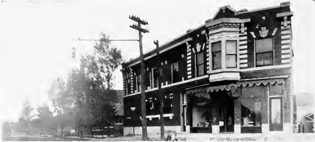
C. MATSON, DAIRY PLANT AND ICE CREAM MANUFACTORY
