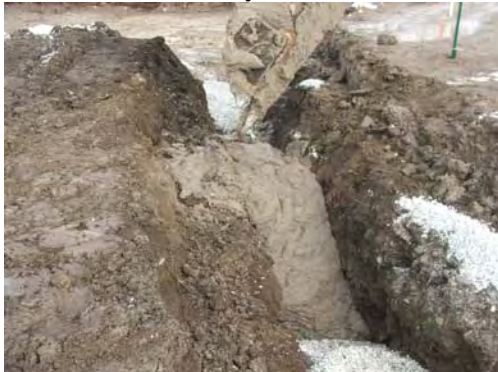
Repair slurry wall at 3" FM pipe location.
