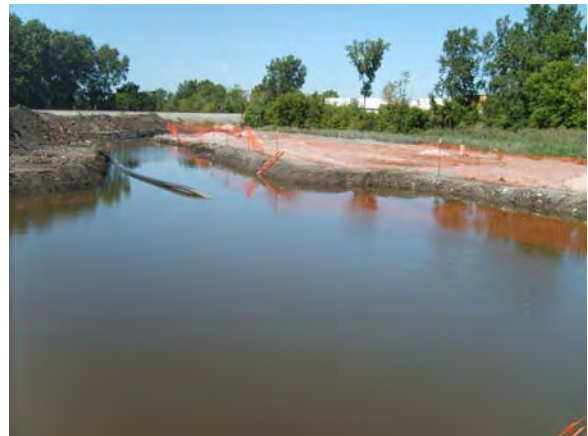
Central sump excavation looking west.
