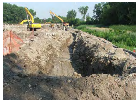
Structural barrier wall
