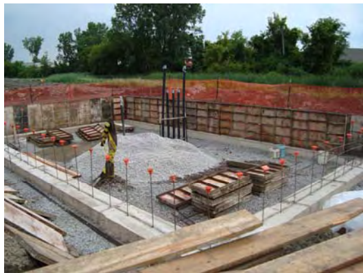
Stone for the floor sump
