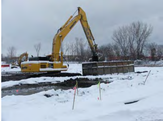
Backfill being mixed and placed into slurry trench.
