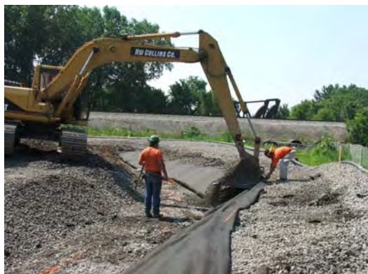
Excavating for structural barrier wall
