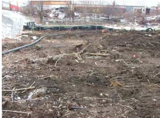
Cleared Northwest corner of site, RR property.
