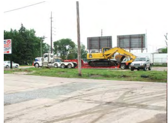
Demobilizing of Envirocon's equipment
