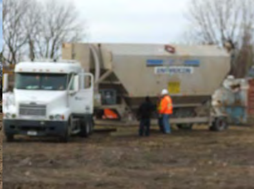
Envirocon begins to set up batch plant.
