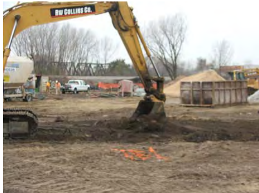
Pre-trenching for slurry wall.
