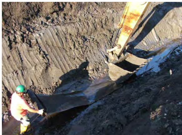
Geotextile 315ST being installed in collection trench #1
