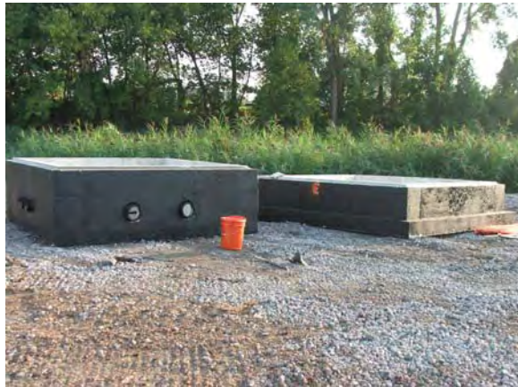
Central sump prepared for placement into excavation.
