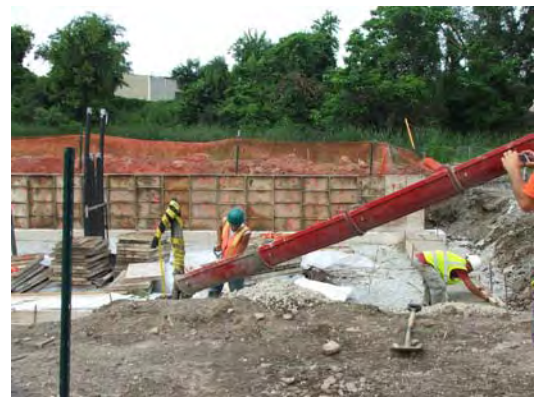
Workers repairing spreader
