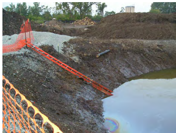
View of central sump excavation looking south.
