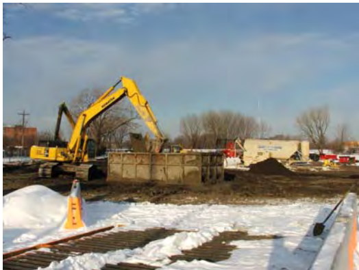
Mixing of backfill for slurry trench.
