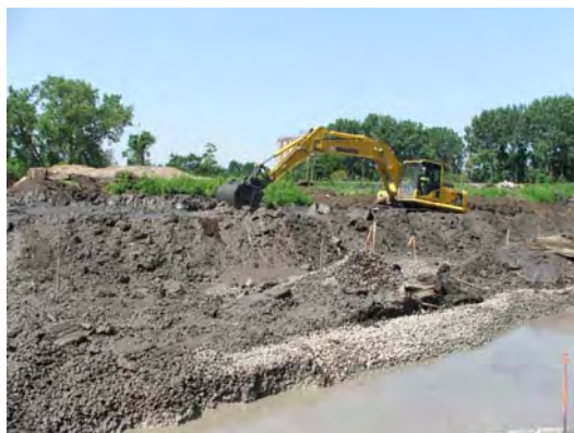
Loader mixing slurry with soil
