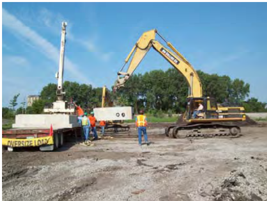
RW Collins unloading central sump sections
