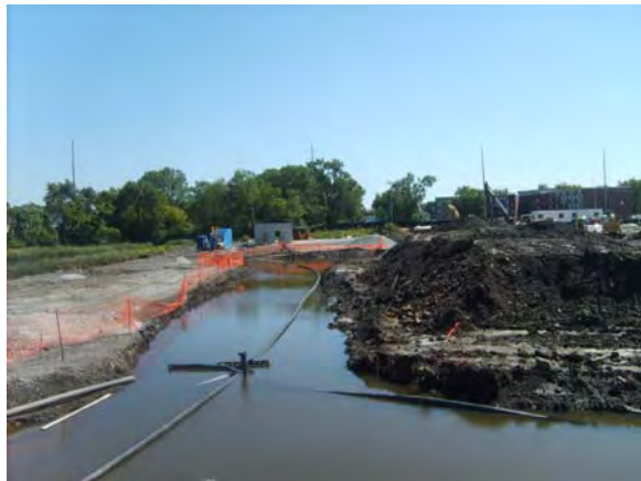
View of collection trench #1 looking east.
