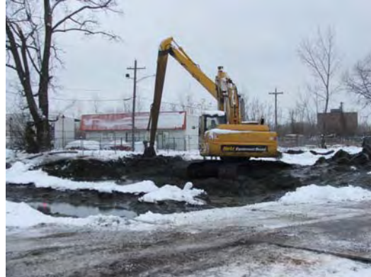
Slurry wall excavation and backfill mixing.
