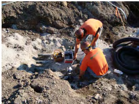
RW Collins performing field pressure check
