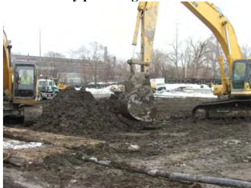
Mixing of backfill for slurry trench.
