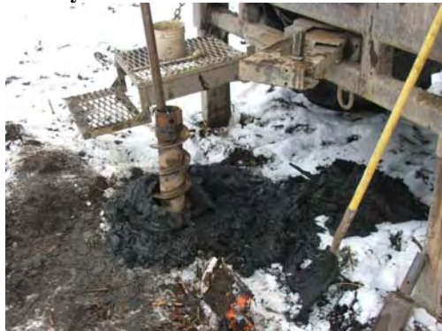
Test borings along Northern alignment.
