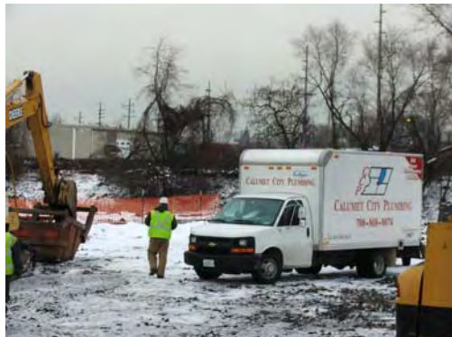
Calumet City plumbing arrives.
