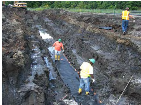
RW Collins placing geotextile material in trench #1.
