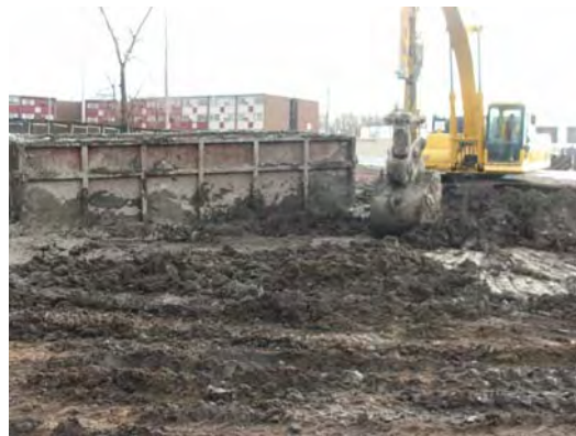
Excavator mixing backfill for use in slurry wall.
