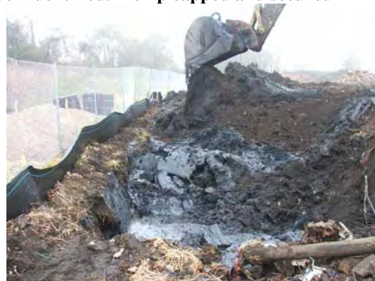
Continued removal of debris/tires.
