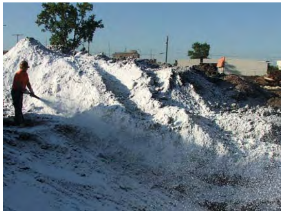
Foaming performed on excavation.
