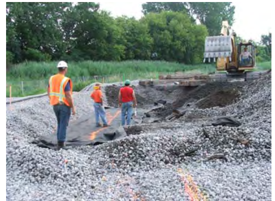
Rw Collins finishing the final stage of the North wall alignment
