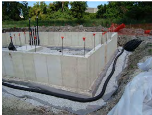
Focus placing drain pipes on outside of treatment building
