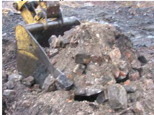
Brick and debris fill inside ring structure.
