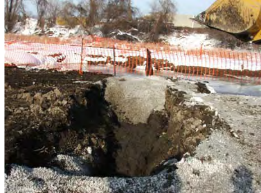
RW Collins Slurry wall repair for 2" water main.
