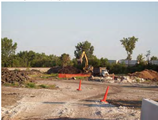
Soils for disposal being loaded
