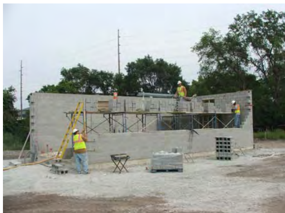
Colvin constructing block treatment building.
