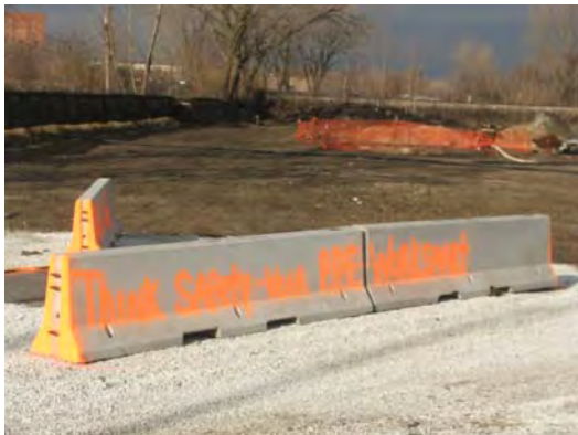
Decon station complete and marked.
