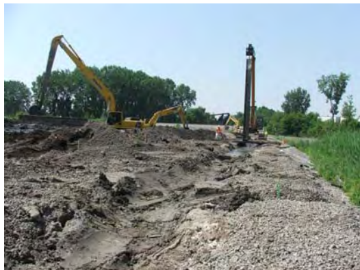
Placing the I beam barrier structure
