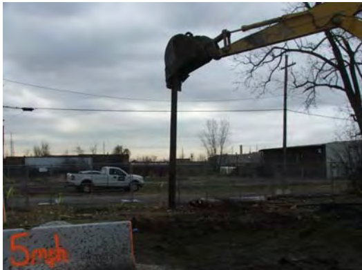
Removal of pole for slurry wall construction.
