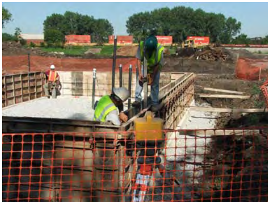
Focus performing quality assurance before pouring concrete
