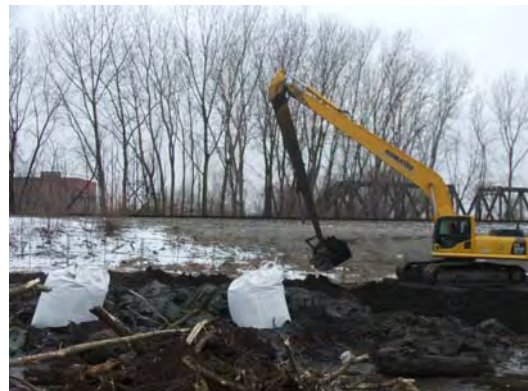
Excavator digging slurry trench.
