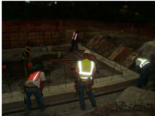
Focus removing forms from Spreader and forming the footer walls
