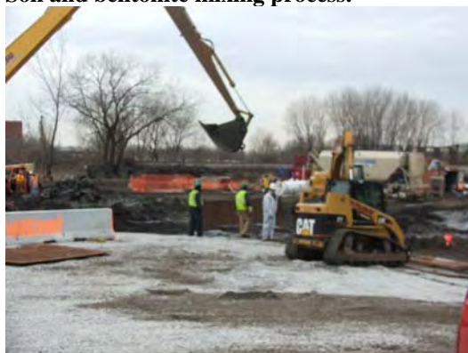
Rw. Collins installing road plates for bridge across slurry.
