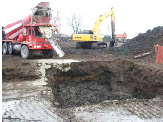
Concrete truck off loading cement for soil stabilization.
