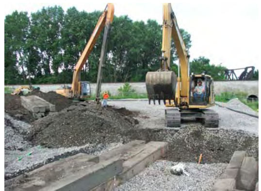
Collins/Envirocon working together pre-trenching
