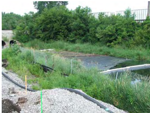
Rw Collins installed 120 ft oil absorbent boom
