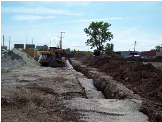
RW Collins preparing electric trench for Focus.
