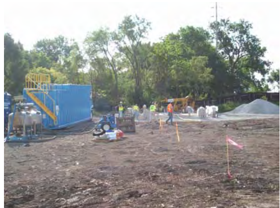
Focus setting up mortar work.
