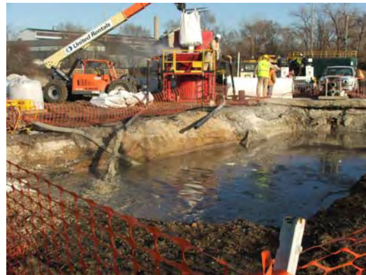
Envirocon beings to premix slurry.
