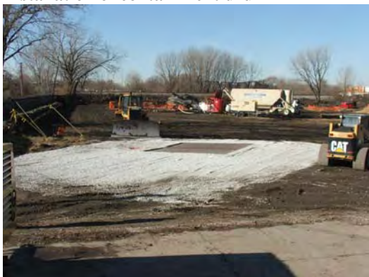
Decon station under construction.
