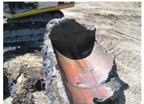
RW Collins uncovers UST Saddle
