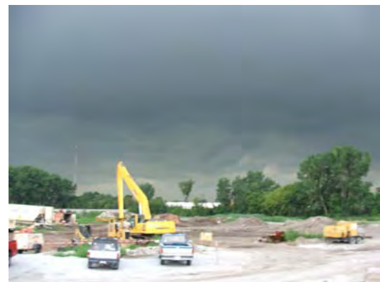
Strong storm passed over site
