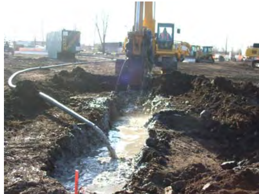
Slurry wall trench begins to fill.
