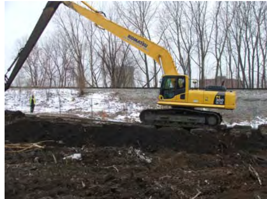
Slurry wall construction to from 1+90 to 1+60.
