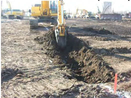
First ground broken in construction of slurry wall.
