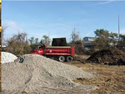
Site grading in preparation for slurry wall.
