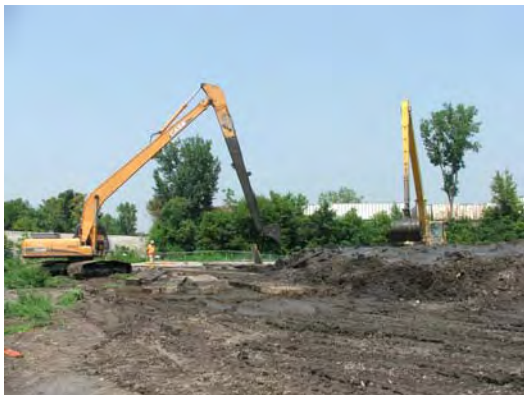
Excavators mixing soil and slurry to form mud
