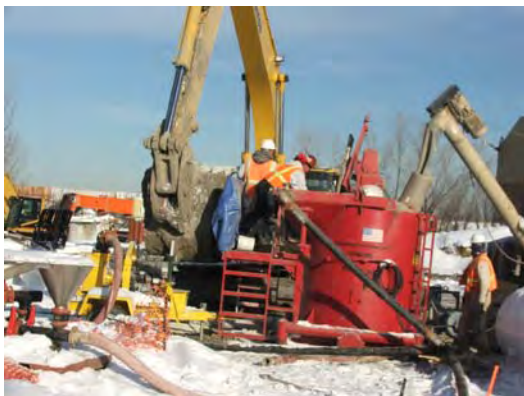
Envirocon batch plant shuts down due to clogging. Soil shear strength testing along northern alignment.
