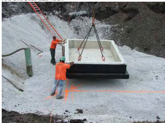
Crane setting central sump structure in place.
