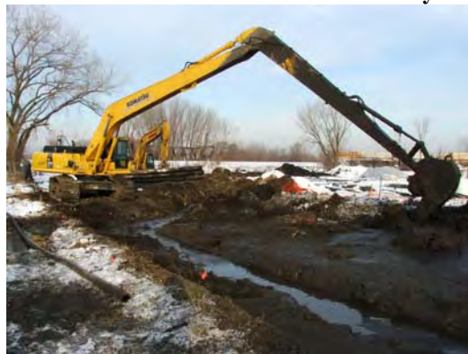
Trench being further cleaned and bad slurry removed.
