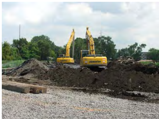
Excavators processing soils/slurry to mud
