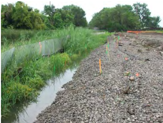
Silt fence inspected after storm, ok.
