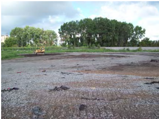
RW Collins grading site.
