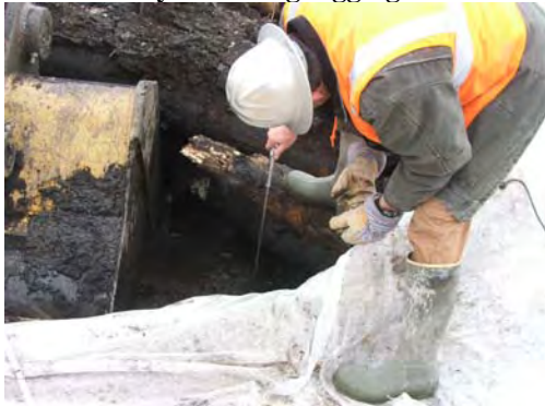
Shear vane testing in the Northern test pits.
