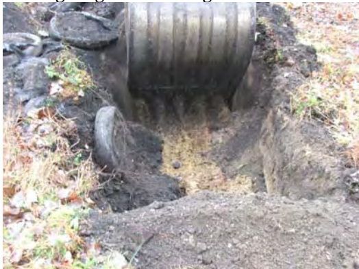
Test pitting along west fence.
