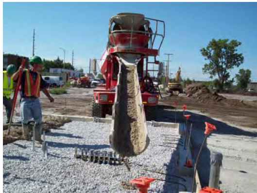
Focus pouring concrete for floor of treatment building.
