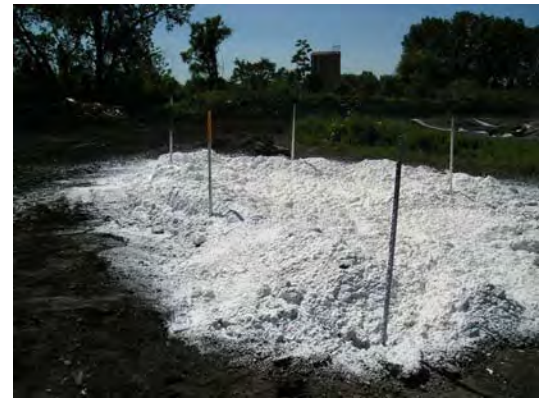
RUSTMAR odor control foam placed on top of tar well
