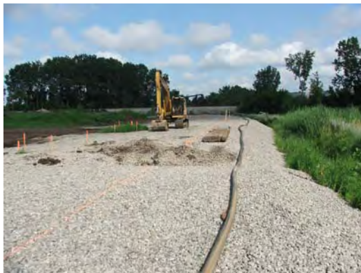
Rw Collins prepping slope for geotextile wrap.
