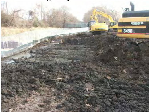
Excavators pulling back the soil from the river.
