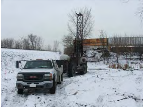
Earth Exp. on site to perform test borings.
