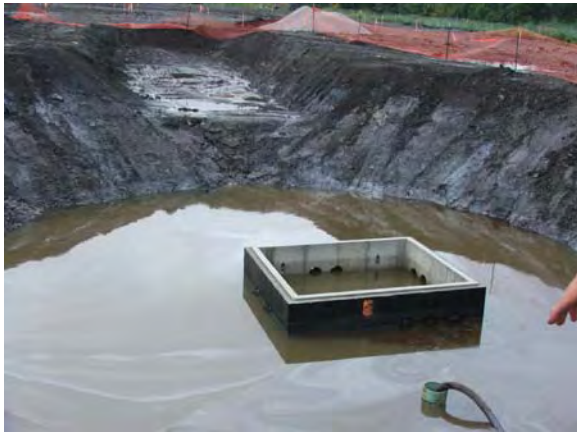
Central sump area being pumped to remove water.
