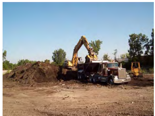
RW Collins loading soil into trucks for disposal
