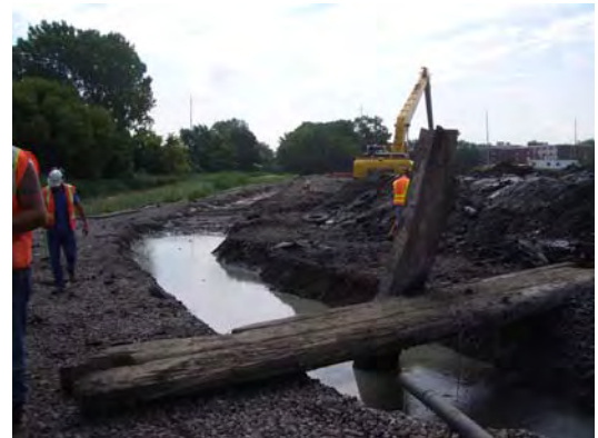
Structural wall installation at STA 1+25
