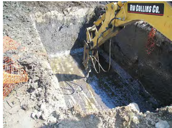
Punching holes in bottom of tar well structure.
