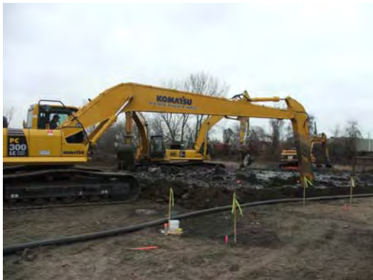
Construction of slurry wall begins from 11+10.
