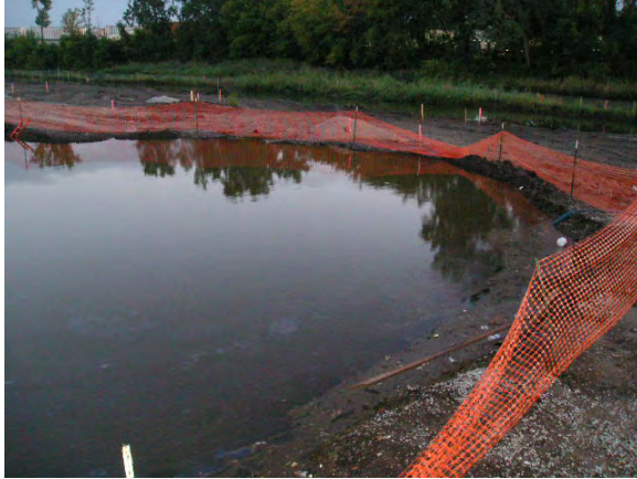
Central sump after main rain event.
