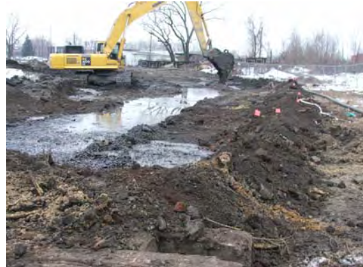
Construction of slurry wall trench from Sta. 2+50 to 1+90.
