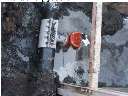
2" water main tap.
