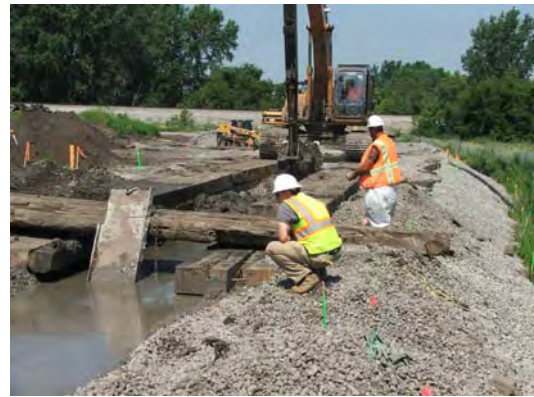
Crew measuring depth of structural barrier wall
