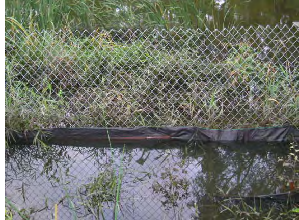
Northern fence line-erosion control still intact.
