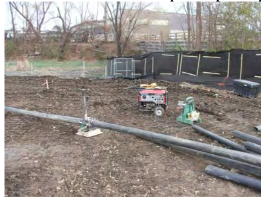
Envirocon continues setting up equipment.
