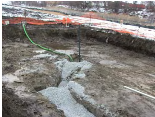
Plumbers back filling trench with stone.
