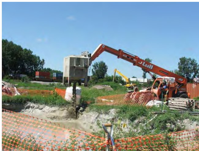
Filling slurry pond with cement to harden
