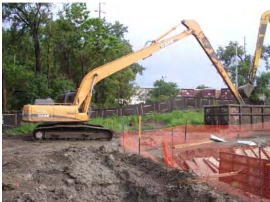
Excavators repairing structural wall at STA 7+56
