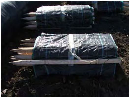
Reinforcing fence arrives.
