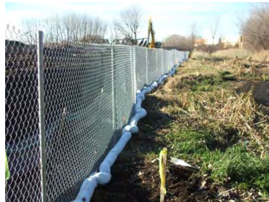
Installation of oil boom along river.
