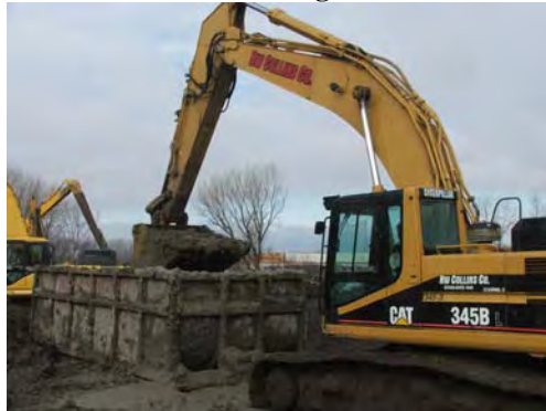
Slurry from Envirocon mix box used for repair.
