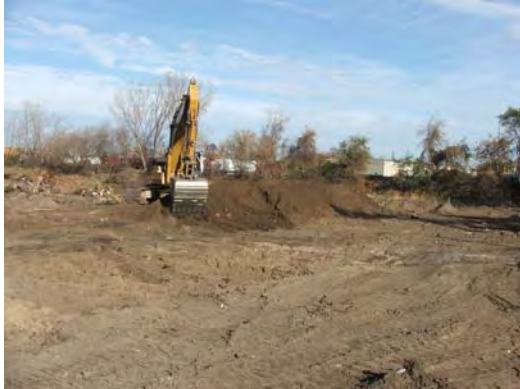
Continued site grading.
