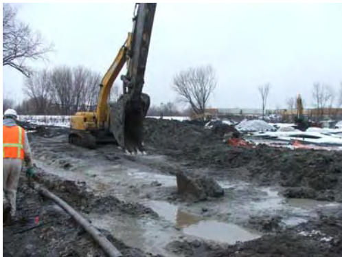
Slurry wall excavation at 6+40.
