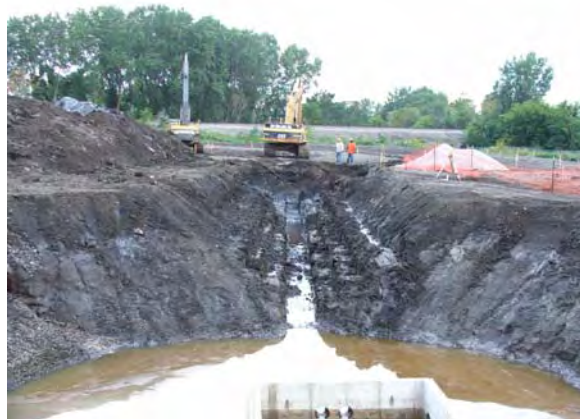
Collection trench#1 excavated to manhole #1.
