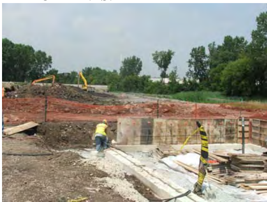
Diamond saw cutting footing spreader
