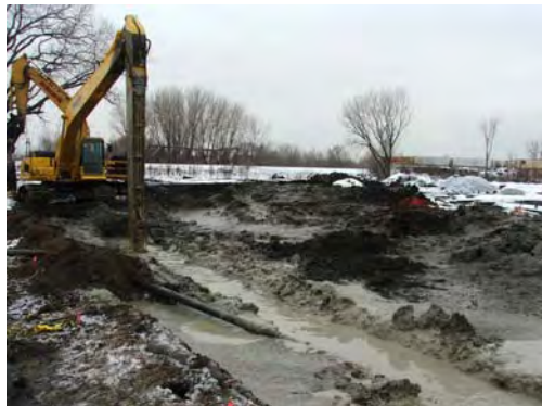
Slurry wall construction from 7+00 to 6+40.
