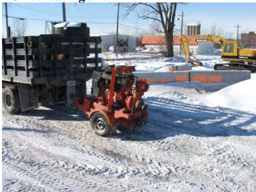
Godwin pump leaving site.
