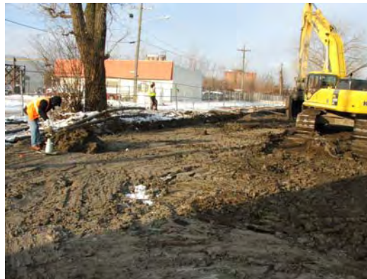
Continued installation of backfill into slurry trench.
