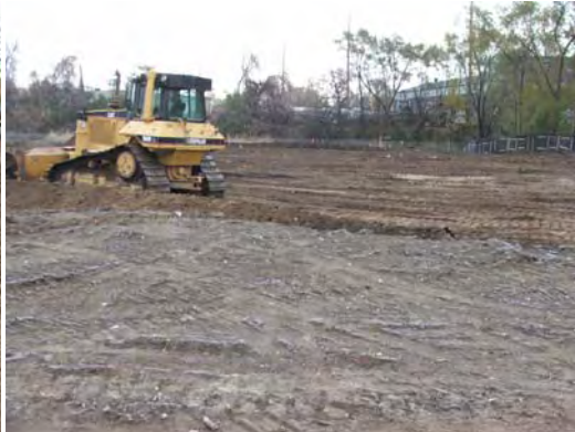
Continued site grading.
