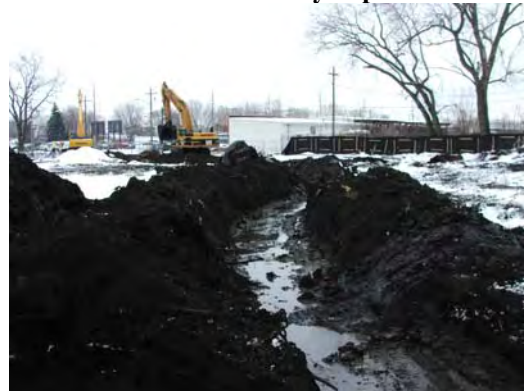
Slurry trench looking South.
