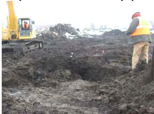
Envirocon test pitting.
