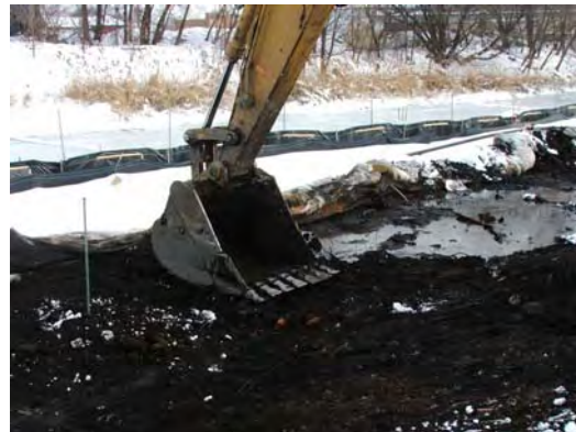
RW Collins backfilling Northern bench in 1 foot lifts.
