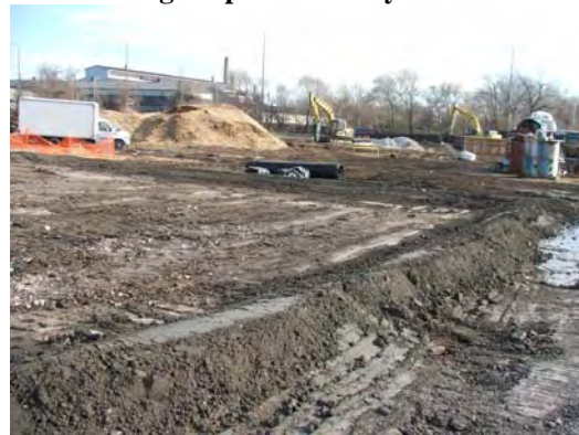
Burm constructed around Soil stockpile area.
