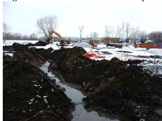
Trench to direct waste slurry to pond.
