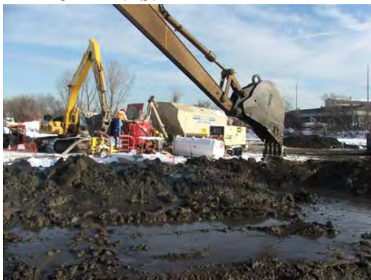
Back filling of trench at STA. 7+50.
