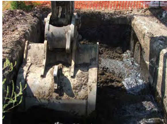
Drying out sludge at the bottom of the tar well.
