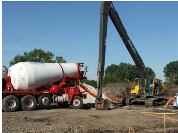
Excavator used to transport concrete into central sump.
