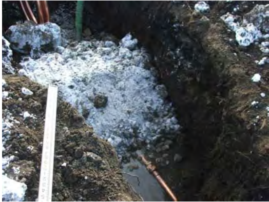
Pipe dam in 2" water main trench.
