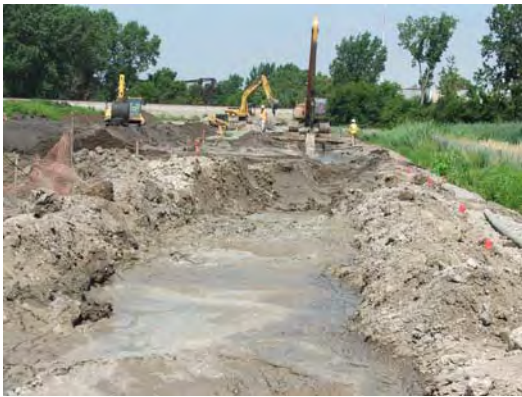
Excavating for structural barrier wall
