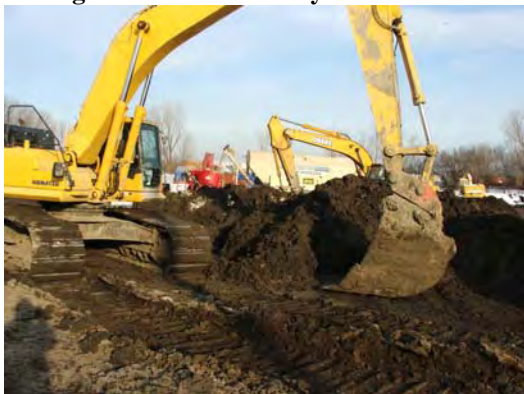
Envirocon mixing fresh bentonite slurry mix.
