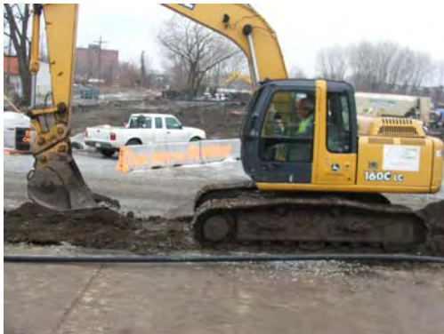
Calumet City Plumbing digging trench for 3' pipe.
