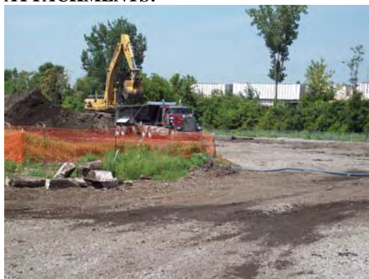
Soils for disposal being loaded.
