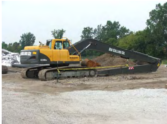
Longstick arrives to help with excavation of trench.
