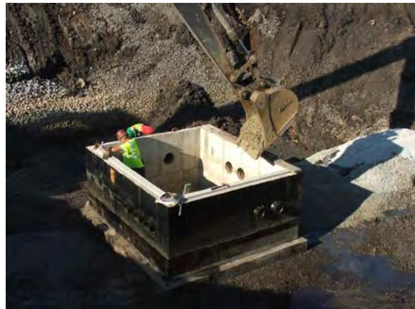
Concrete work in central sump.
