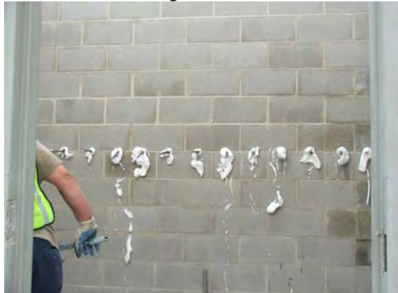
Foam injected into block walls of treatment building.
