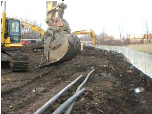
Excavators begin to pull soil back from river
