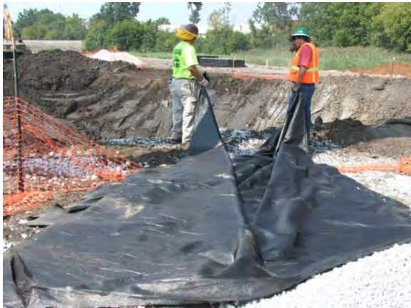
Fabric being prepared for sump.
