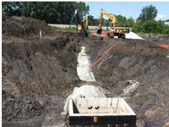
RW Collins installed clay pipe dam as per spec in trench #1.
