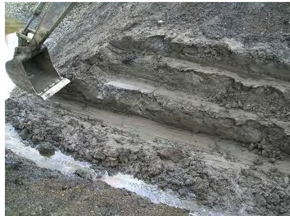
Work on trench#1 with longstick excavator.
