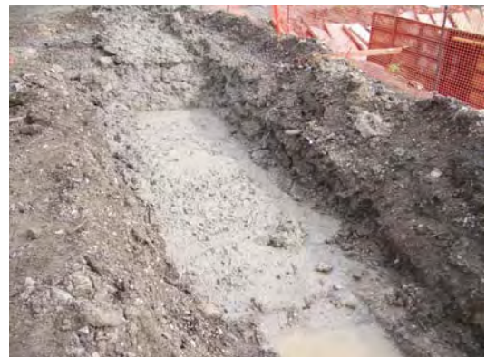
Repair of structural wall at STA 7+56
