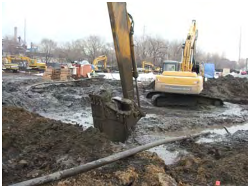
Construction of slurry wall between 5+80 and 4+60.
