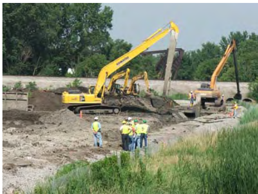
Excavating for structural barrier wall (IDEM site visit)
