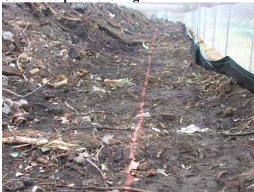
Continued removal of debris/tires.
