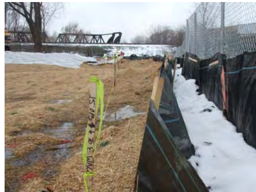
Line of stakes on North alignment.
