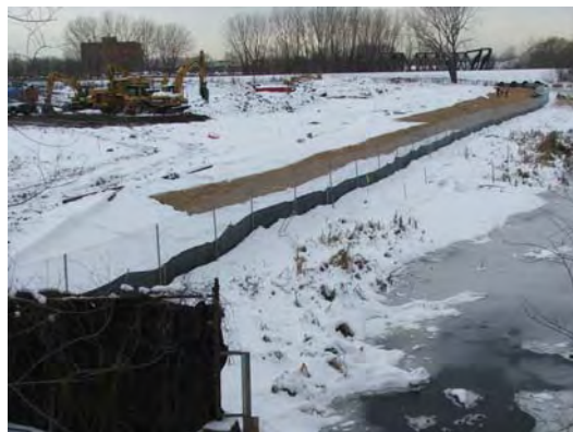
Northern slope of site with erosion control installed.
