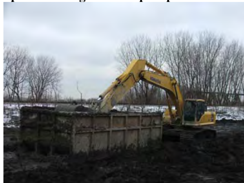
Construction of slurry wall.
