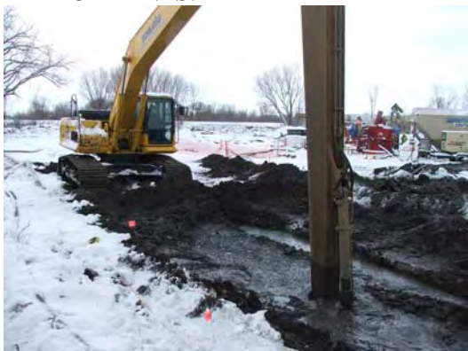
Slurry wall construction from Sta 8+00 to 7+00
