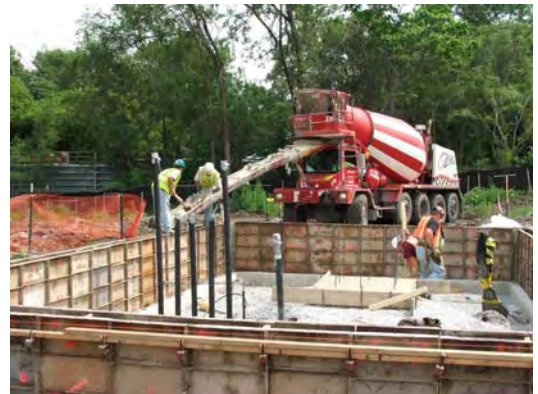
Focus pouring concrete for walls
