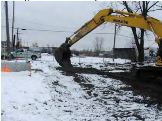
Placement of backfill into existing trench.
