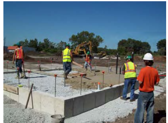
Focus leveling concrete floor of treatment building.
