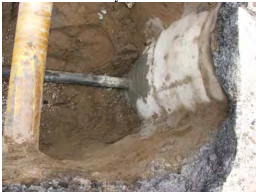
Connection to sanitary catch basin completed.
