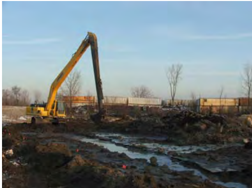
Excavation of slurry wall trench at sta 3+00 to 2+50. Pipe dam being installed per spec.
