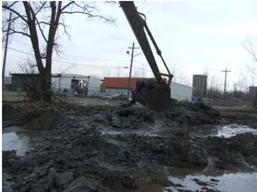
Slurry trench under construction.
