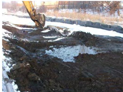
Backfilling bench from 1+50 to 6+50.
