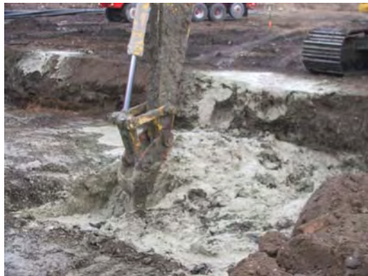
Envirocon mixing cement & soil for stabilization.
