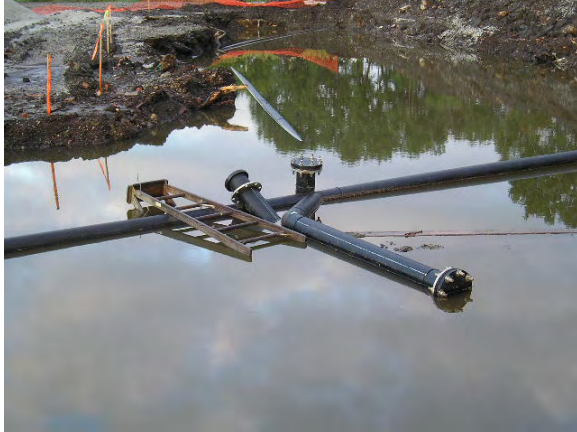
6" HDPE piping at location of Manhole #1.
