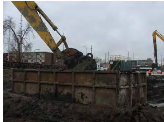
Mixing backfill to place in slurry trench.
