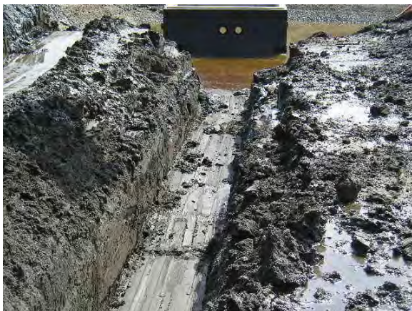
View of trench #1-Looking west to east.
