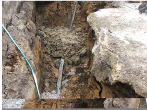
Excavation of slurry wall trench at sta 3+00 to 2+50. Pipe dam being installed per spec.
