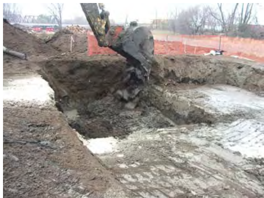
Envirocon excavating final 15'X15' stabilization area.
