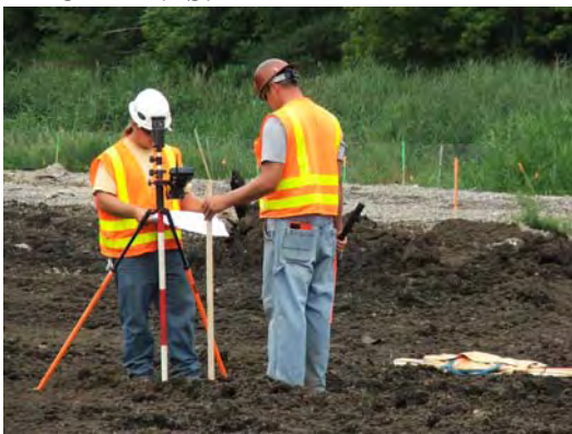
W. T. Surveyors surveyed final settlement points
