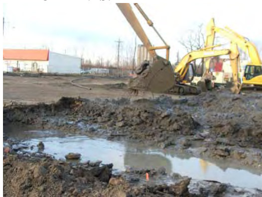
Continued construction of slurry wall from Sta.10+00 to 9+10.
