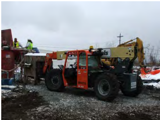
Making new batch of slurry.
