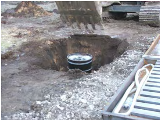
Installation of containment drum
