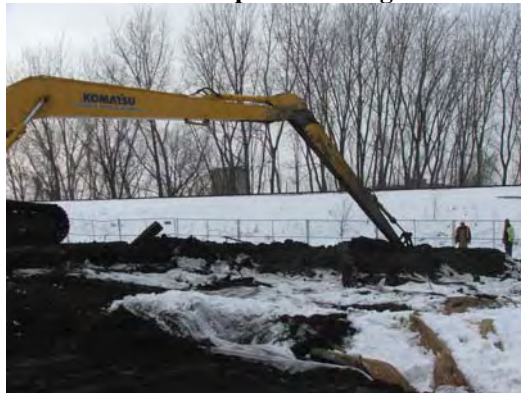
Envirocon test pitting.
