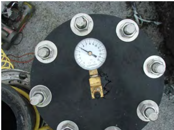
Low pressure Air testing done on 6" HDPE piping.
