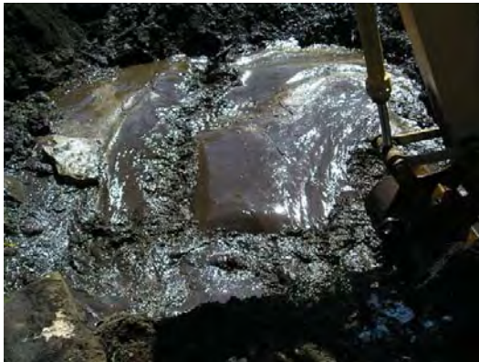
RW Collins uncovers UST
