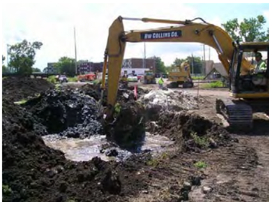
RW Collins performs exploratory excavations
