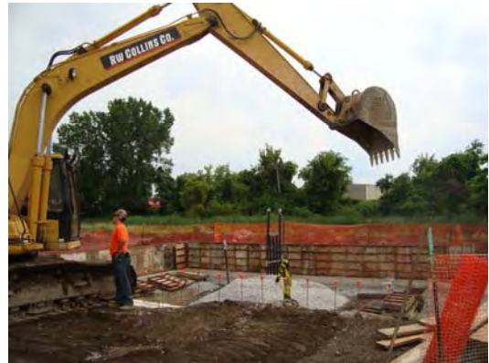
Collins is adding stone for the bottom grade of floor sump
