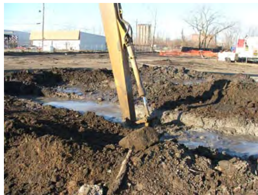
Construction of slurry wall.
