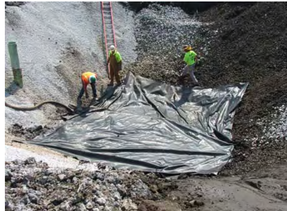
Stone on sides of excavation and fabric on bottom.
