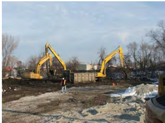
Slurry wall trench construction wrap up.
