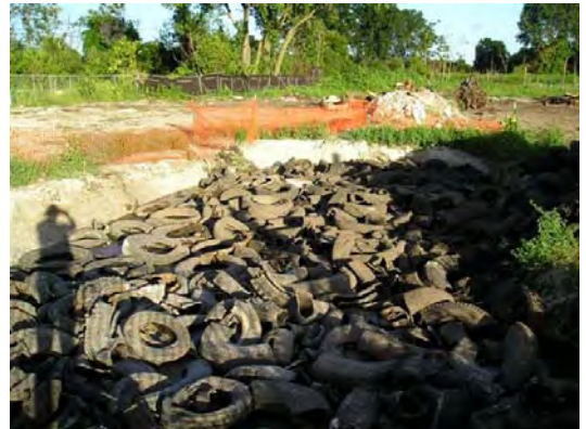
RW Collins burying tires, slag and other debris
