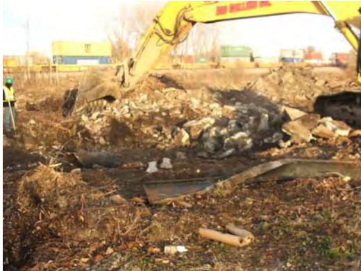
Continued removal of concrete.
