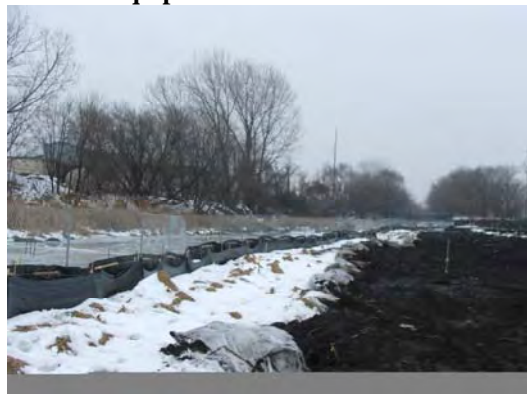
View of silt fence from Northwest corner.
