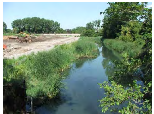
RW Collins removing debris from north side of property.
