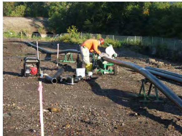
RW Collins working on HDPE pipe fusion.
