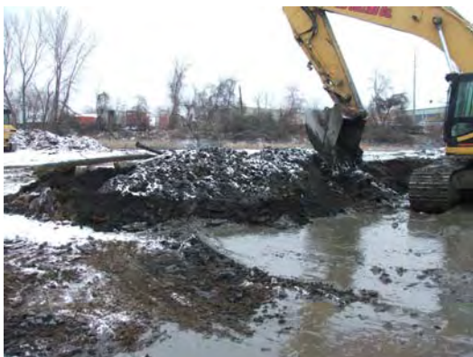
Peat excavated from trench, stockpiled and berm placed around it.
