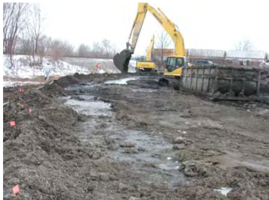
Construction of slurry wall trench.
