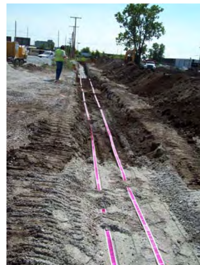
RW Collins laying metallic tracing tape for pipe runs
