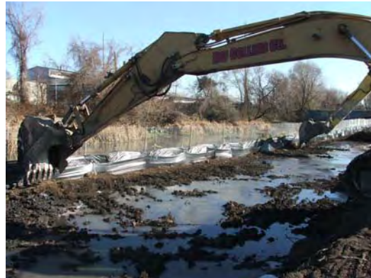
Grooming bench for erosion control mat install.
