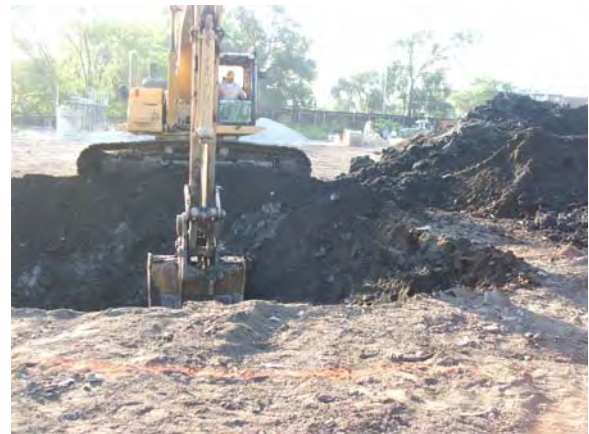
Expanding central sump area.
