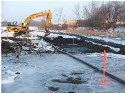
RW Collins backfilling lower bench.
