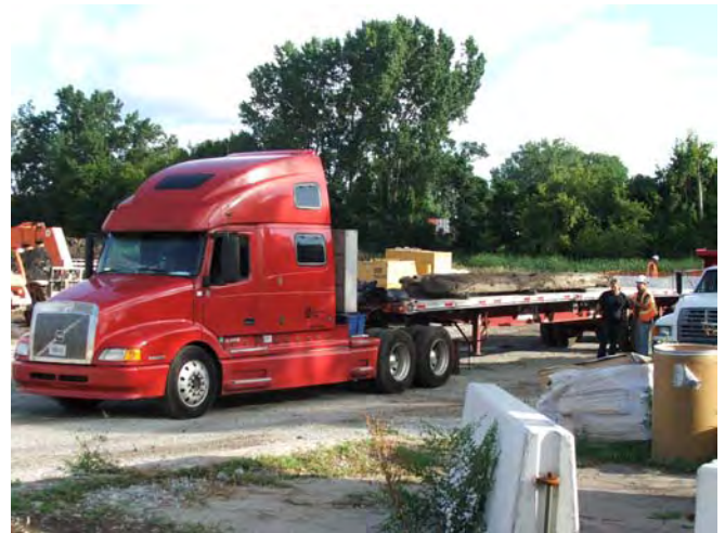
Envirocon loading crane mats on truck
