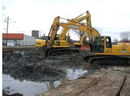
Backfill being mixed for use in slurry wall.
