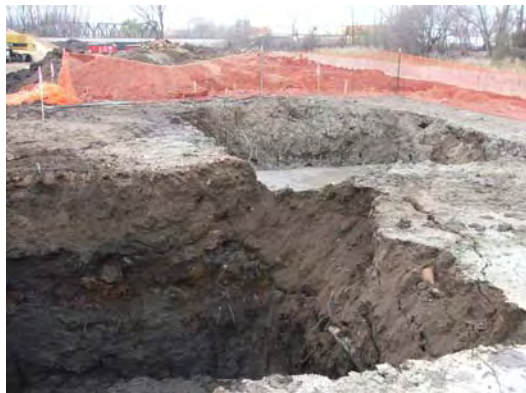
Envirocon Soil stabilization Excavation
