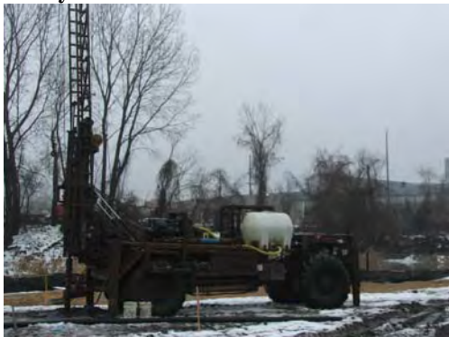
Test borings being performed along North alignment.
