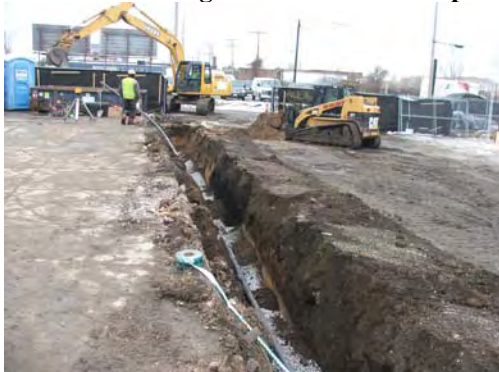
Calumet City plumbing trench with piping.
