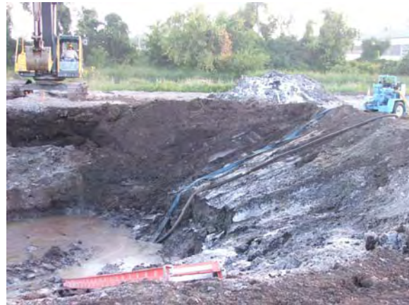
RW Collins continues excavation of sump, and dewatering.
