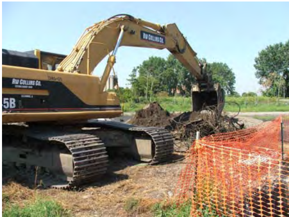
Segregating soil into containment area.
