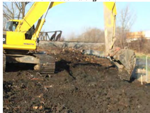
Continued grading of site.
