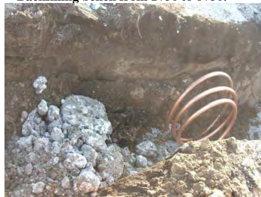
Continued work in 3" main trench.
