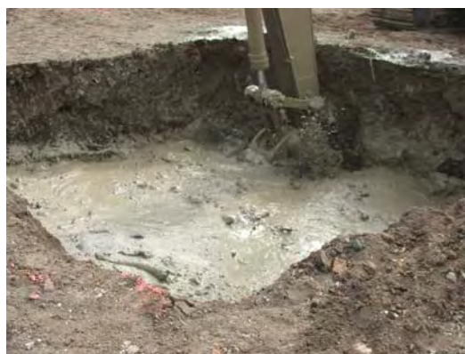
Excavator mixing cement with excavated soils.
