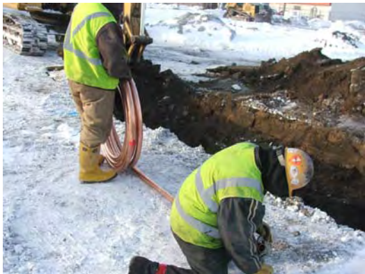
Plumbers working on 2" water main.
