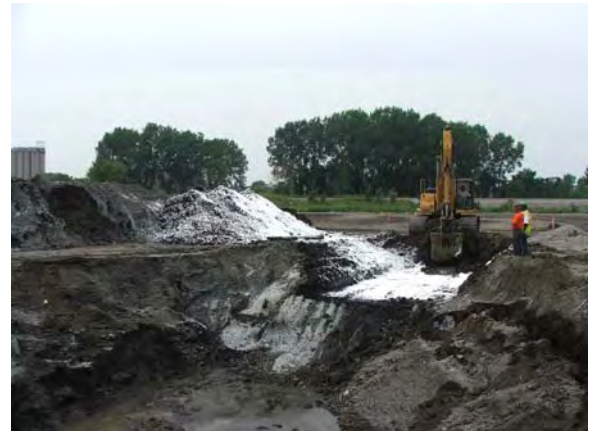
Test pitting to determine soil conditions.
