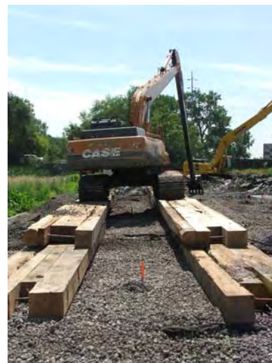
Stacked crane mats in use
