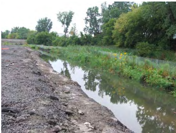
Northern slope flooded due to rain.
