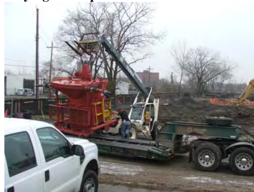
Envirocon continues to set up batch plant equipment.
