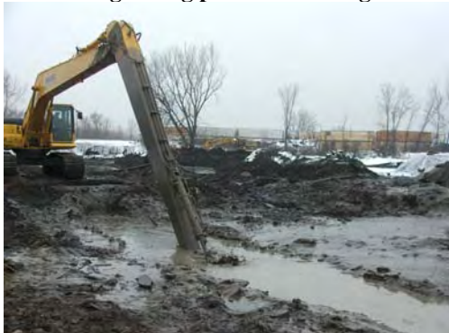
Slurry wall excavation at 5+80.
