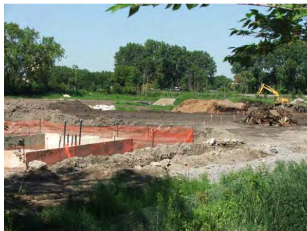
Focus removed forms from building.
