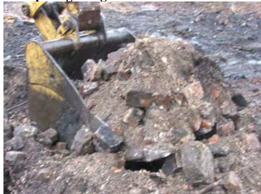
Brick and debris fill inside ring structure.
