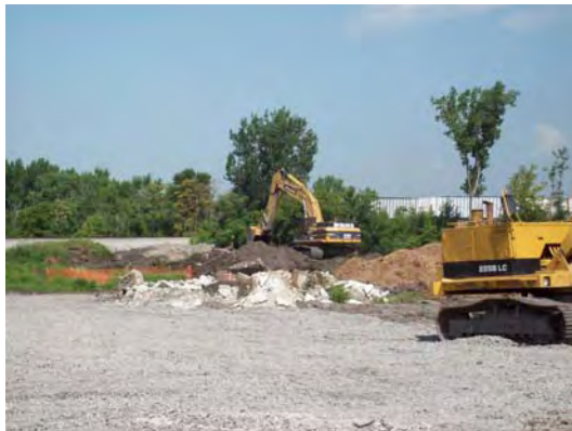
RW Collins separating debris from soil for disposal
