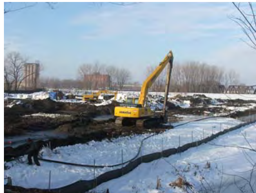
View of North Slope from bridge offsite.
