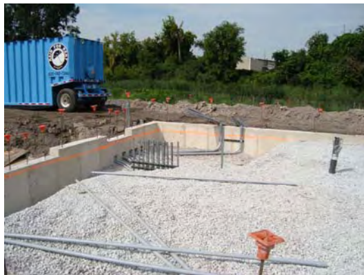
Treatment building backfilled
