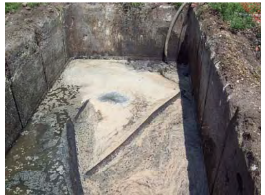
Dewatering tar well for regeneration observation
