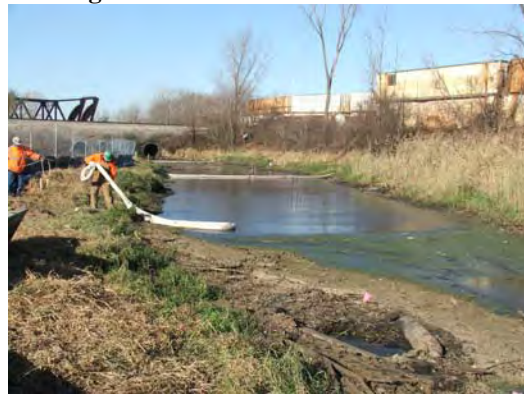
Installation of two booms across river.
