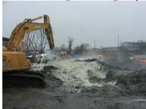
Excavator creating bentonite mixture.
