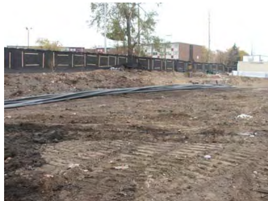
Envirocon Staging HDPE pipe on site.
