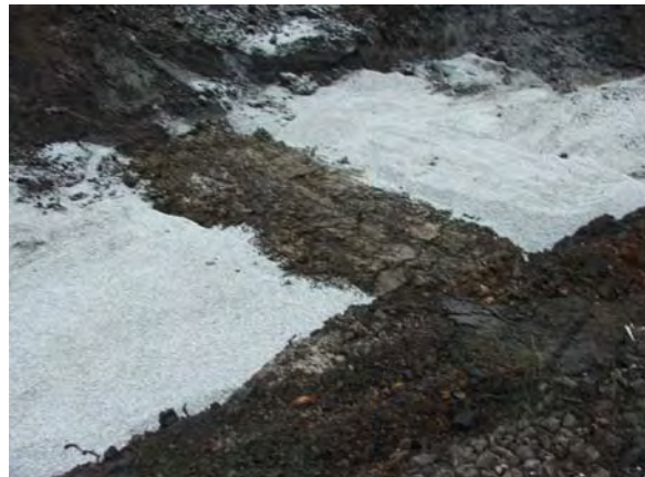
Pipe dam installed in collection trenches #1 and #6.
