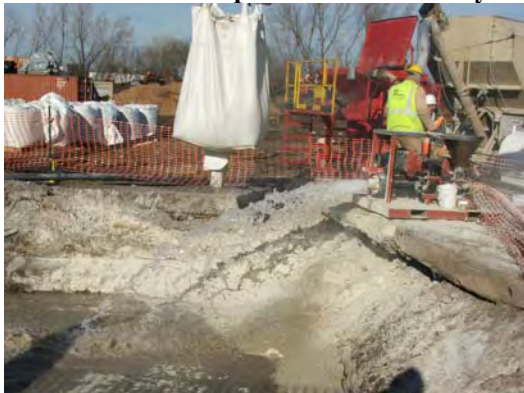
Envirocon begins mixing process.
