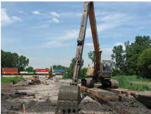
Excavating for structural barrier wall
