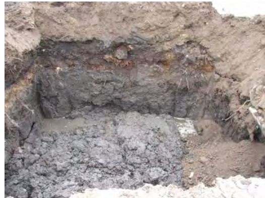
Pre-trenching for slurry wall.
