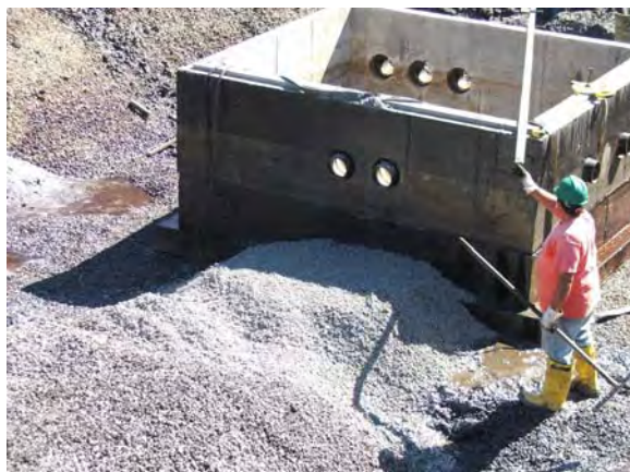
Prep of central sump and placement of stone for HDPE pipes.
