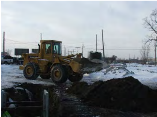
RW Collins grading site.
