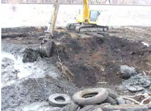
Burming soil for slurry wall.
