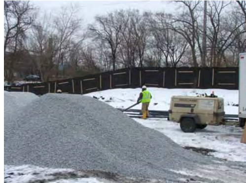
Calumet plumbing back fill for force main.
