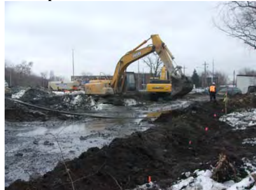
Construction of slurry wall from sta. 4+60
