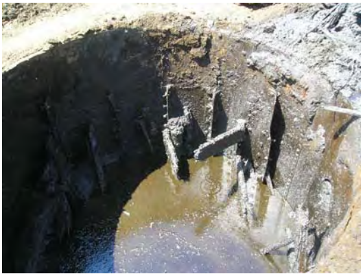
RW Collins located tar well.
