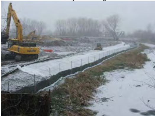
Full view of jute matting along northern boundary.
