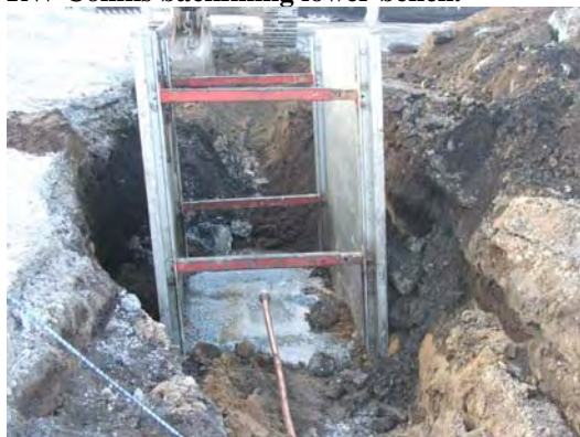
Installation of pipe dam.
