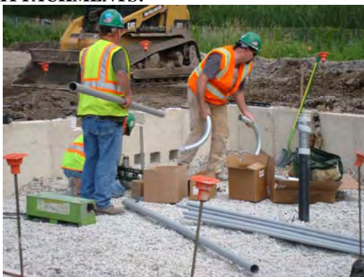
Focus installing conduits
