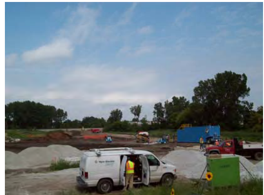
Focus installing conduits
