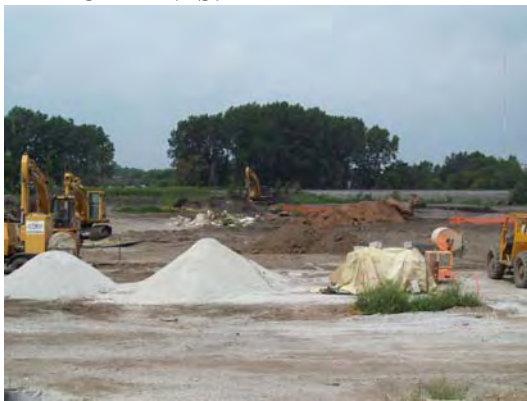
RW Collins grading site
