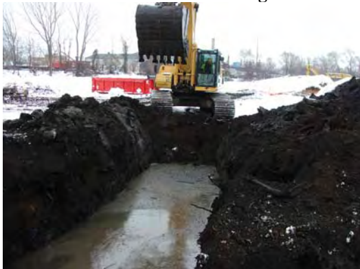
Excavation for waste slurry.
