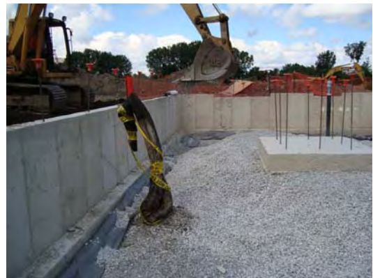
RW Collins backfilling treatment building.
