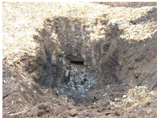
Test pitting for tar well, Trough only structure found.
