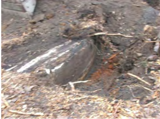
Investigating concrete ring structure.
