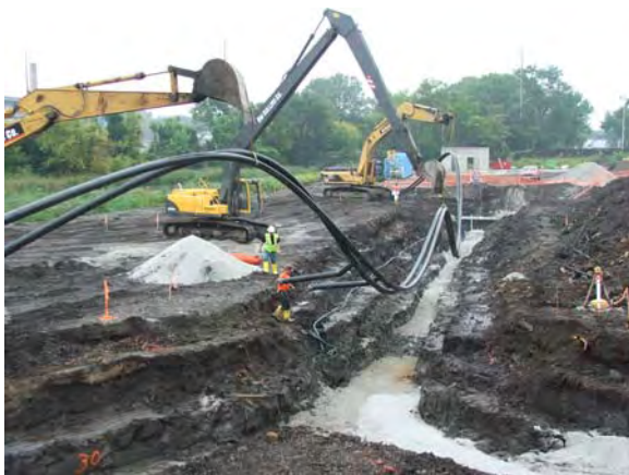
6" HDPE pipe being placed into collection trench #1.
