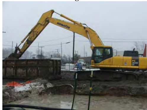
Excavator mixing backfill along slurry excavation.
