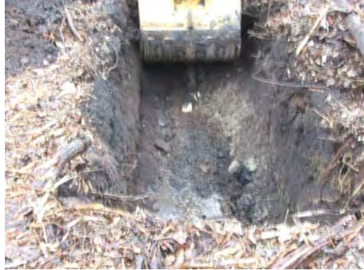
Test pitting along west fence for alternate location.
