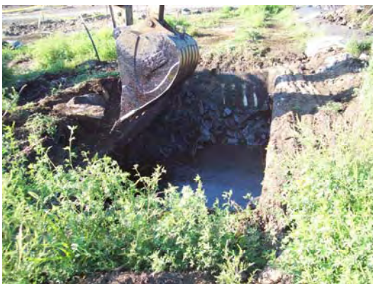
RW Collins removing soil and debris from tar well
