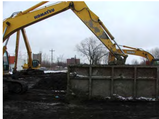
Mixing of bentonite and soil for fresh slurry.
