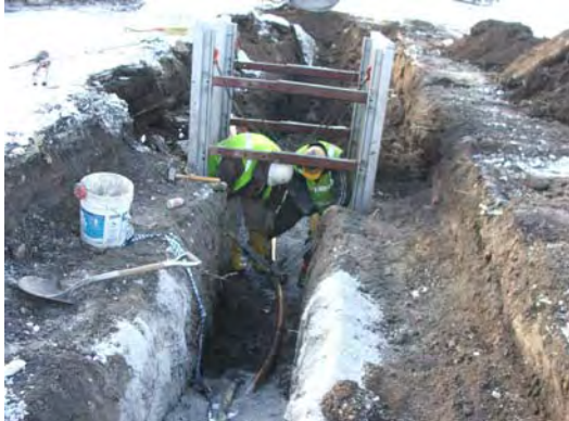
Plumbers working in trench box.
