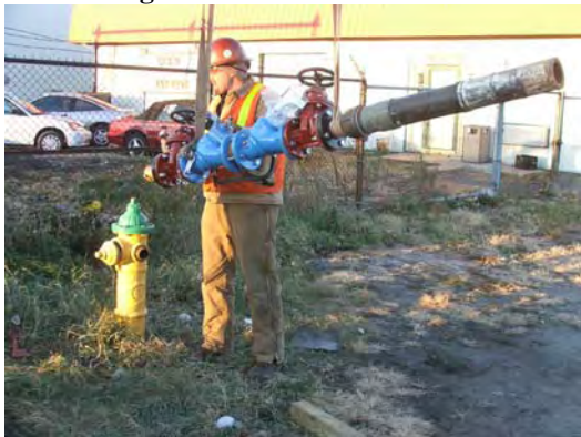
Envirocon connects plant to local water hydrant.
