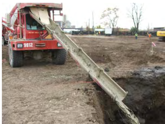
Concrete truck off loading cement mix.
