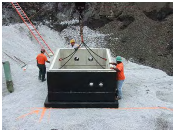
Central sump structure in place.
