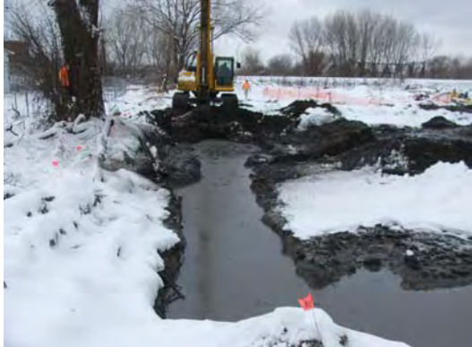
Slurry trench along South property line.
