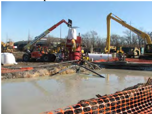
Envirocon continuing to mix slurry at batch plant.
