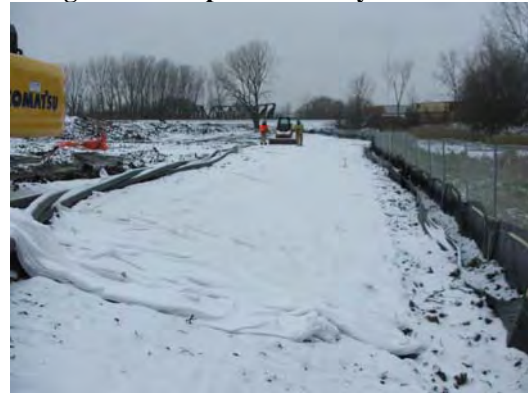
Jute matting to control erosion.
