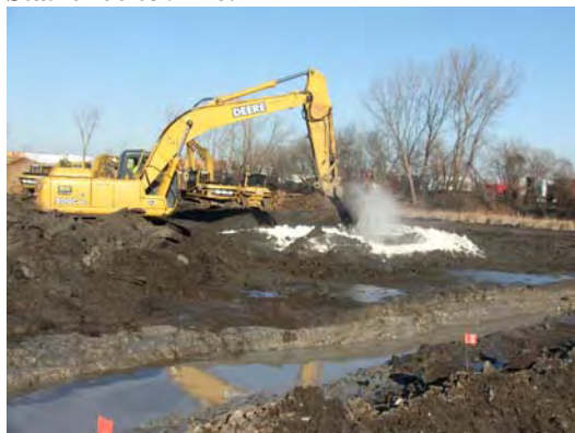
Soil and bentonite mixing process.
