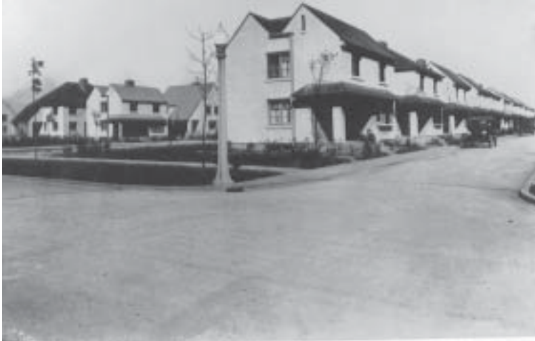
Park Street at Pine Avenue. Note the original cast concrete light post at the corner. When Marktown was first built, the only fences were the two concrete fences on the 500 block of Lilac Street. Note the open porches which actually increased the level of security for each home. Circa 1920.
