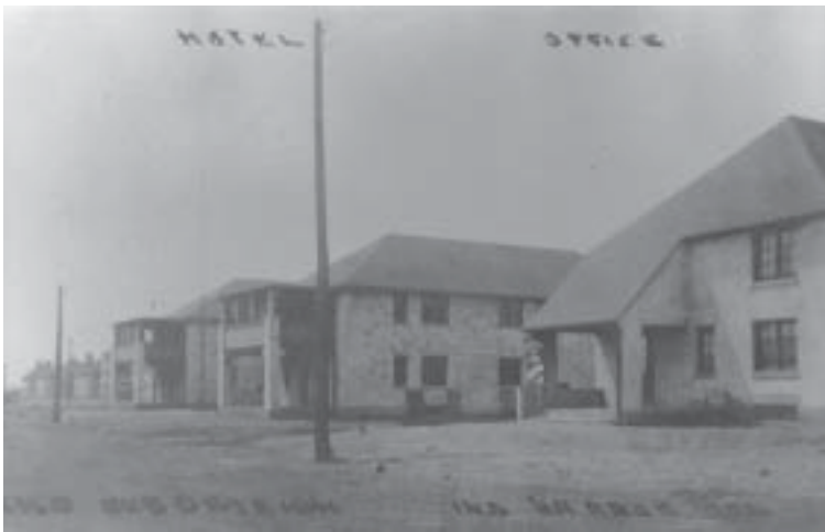
Back when Marktown was new, the primary means of long distance communication was the Post Card. In an early 1917 or '18 postcard the Mark Hotel and the first Post Office/Rental office are depicted here. Note that the finish coat of stucco had not been applied.
