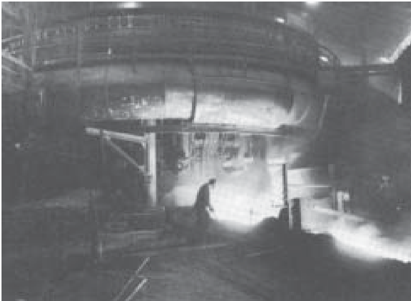
The Blast Furnace was the first step in the steel making process. Here, iron ore is mixed with limestone and coke. The end product is hot metal or pig iron which was then used in the open hearth operations.
