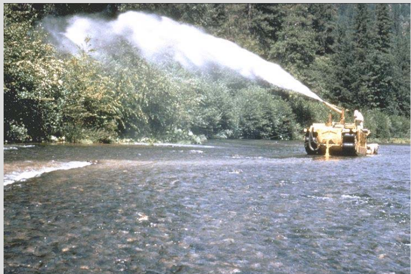
Hydroseeding of a streambank. Source: In Stream Corridor Restoration: Principals, Processes, and Practices (10/98). By the Federal Integrcy Stream Restoration Working Group (FISRWG)
