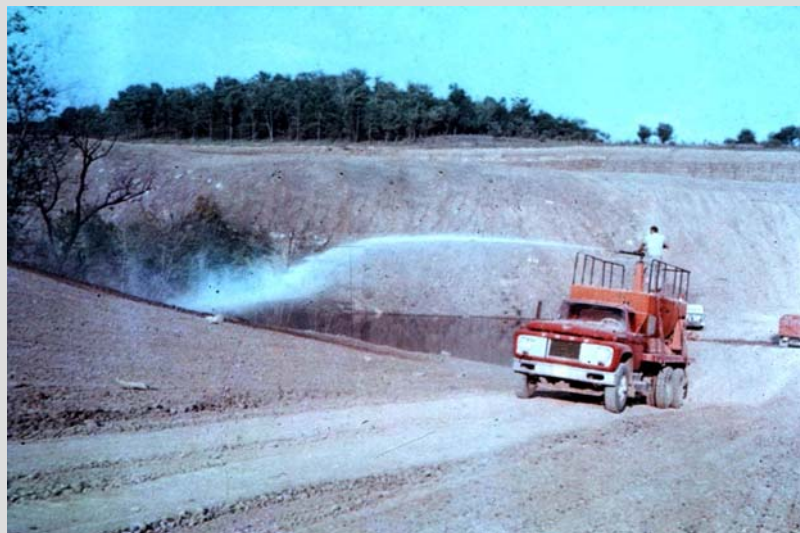
Hydroseeding of a streambank. Source: In Stream Corridor Restoration: Principals, Processes, and Practices (10/98). By the Federal Integrcy Stream Restoration Working Group (FISRWG)
