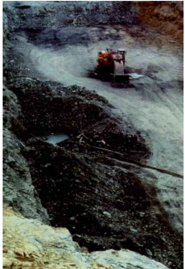
Coal combustion waste fill site where a pump is used to remove ground water.
