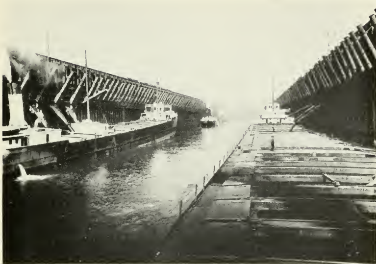
PLATE 3.—A section of the Ore Docks at Duluth showing loading operations in progress, the dock structure, and the loading spouts.
