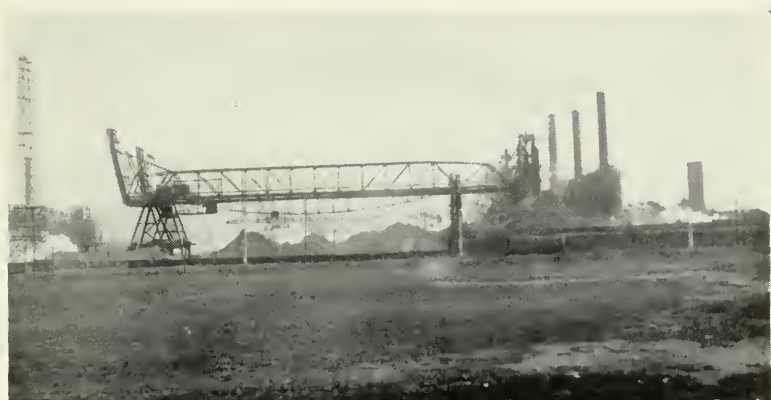
PLATE II.—The Ore Piles, Bridge Conveyors, and Blast Furnaces of the Iroquois Plant, South Chicago.
