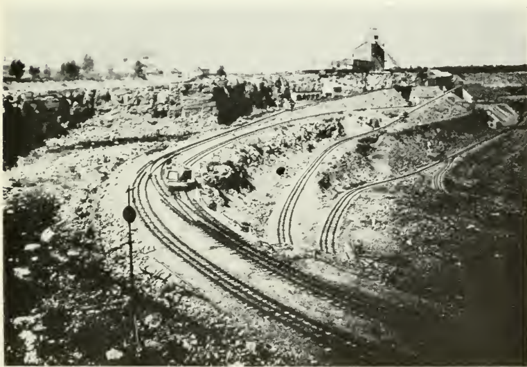
PLATE 10.—A Limestone Quarry at Alpena, Michigan. The picture shows the various levels at which the stone is being quarried, and the series of railroad tracks by which it is assembled at the crusher. The thin overburden, about four feet thick at this point, can be seen clearly at the left of the picture.
