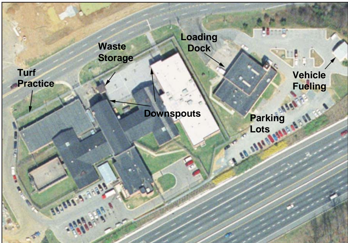
Figure 24: Investigating Potential Storm Water Hotspots
