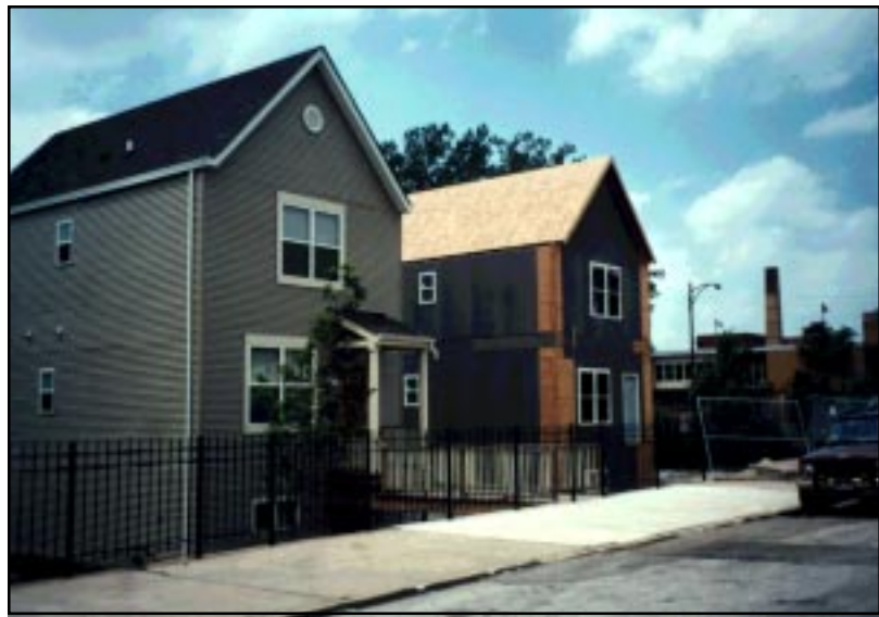
Reinvestment in our community will bring about significant improvement of our housing stock.
