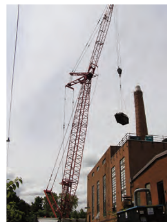
At Smith College, a crane installs components of the new cogeneration system.
