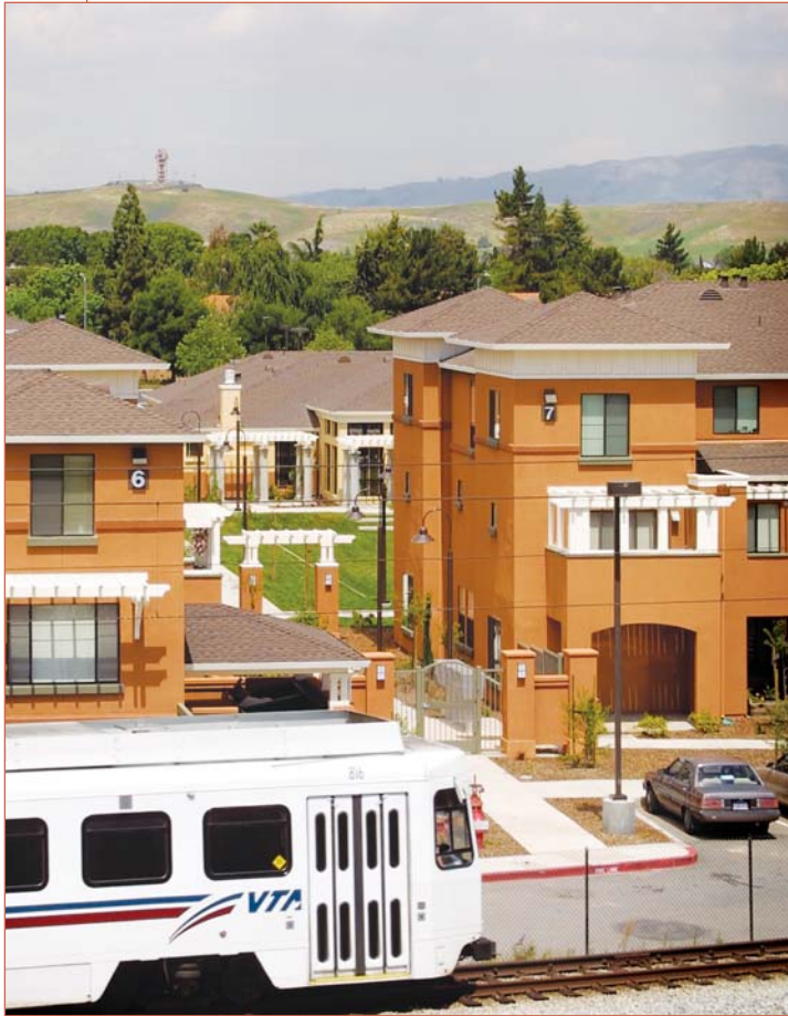
Ohlone-Chynoweth station pioneered both multifamily and affordable housing in a single-family neighborhood in San Jose, CA.
