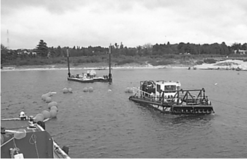
Hydraulic dredging project
