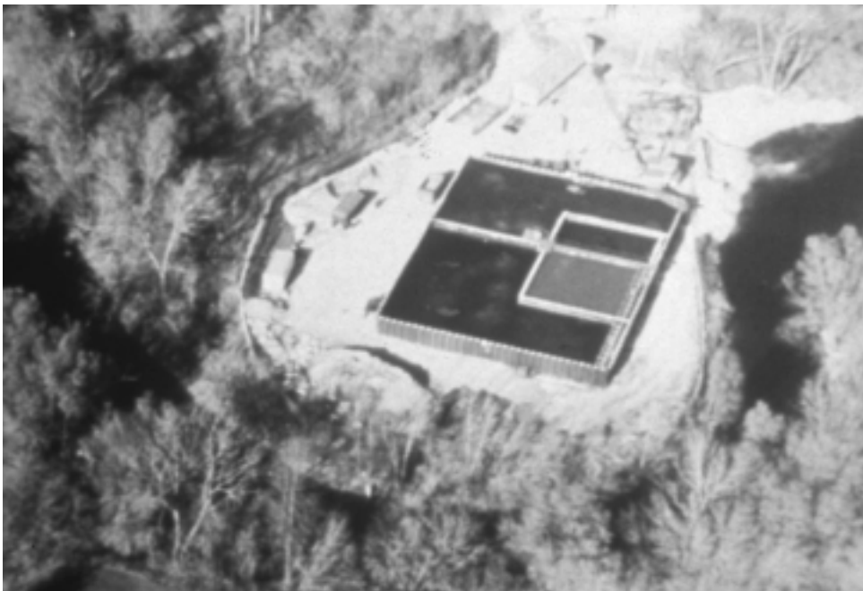
Biological treatment unit at Sheboygan, WI
