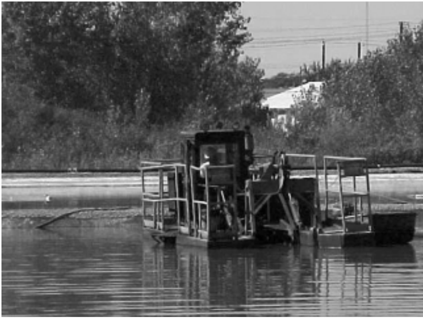
Hydraulic dredge operator on the Fox River
