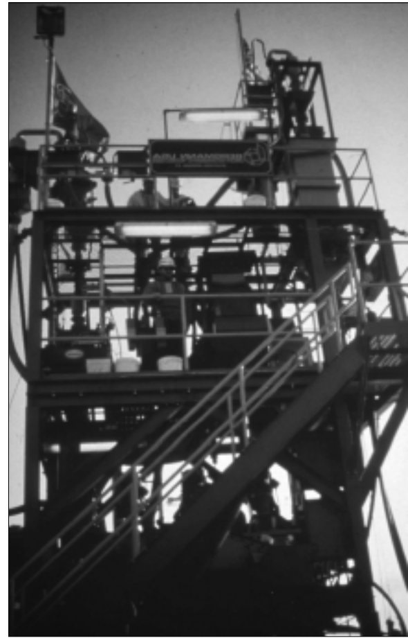
Soil washing process
