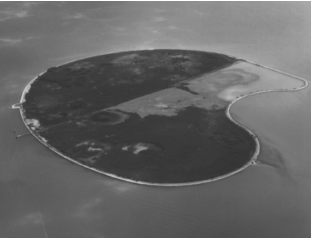
Confined disposal facility in Saginaw, MI
