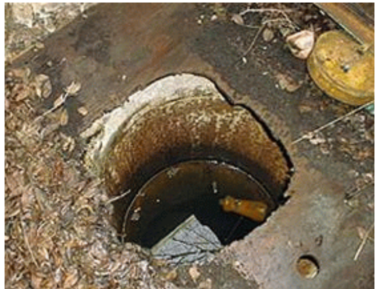
Figure 10. Uncovered abandoned well containing garbage Source: CLOCA, 2005
