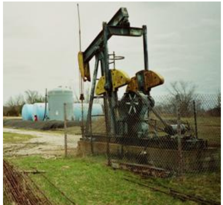
Figure 7. Brine well and storage tanks with secondary containment, Kent Co., Ontario Photo By: D.W. Alley, 2007
