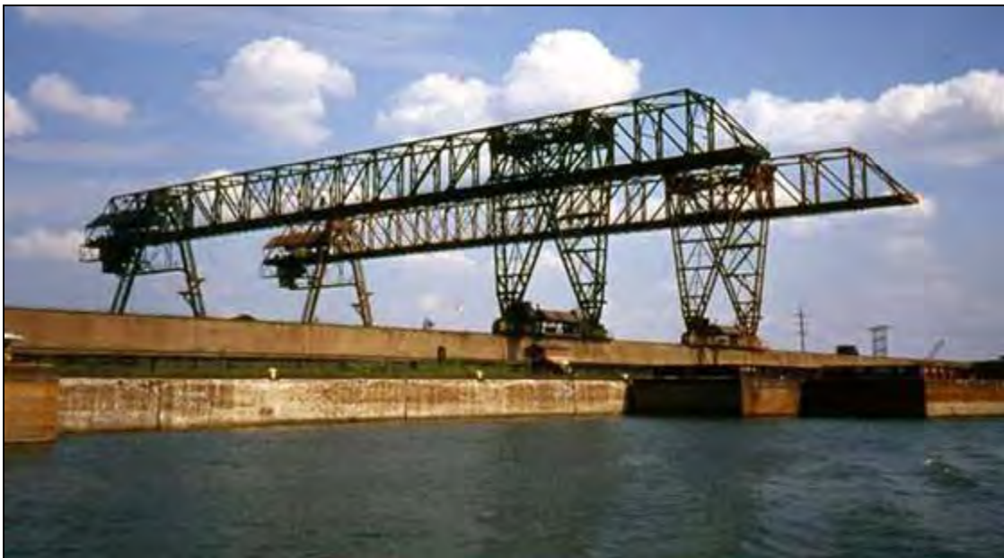
41. Overhead Cranes LTV, 7/29/2004
