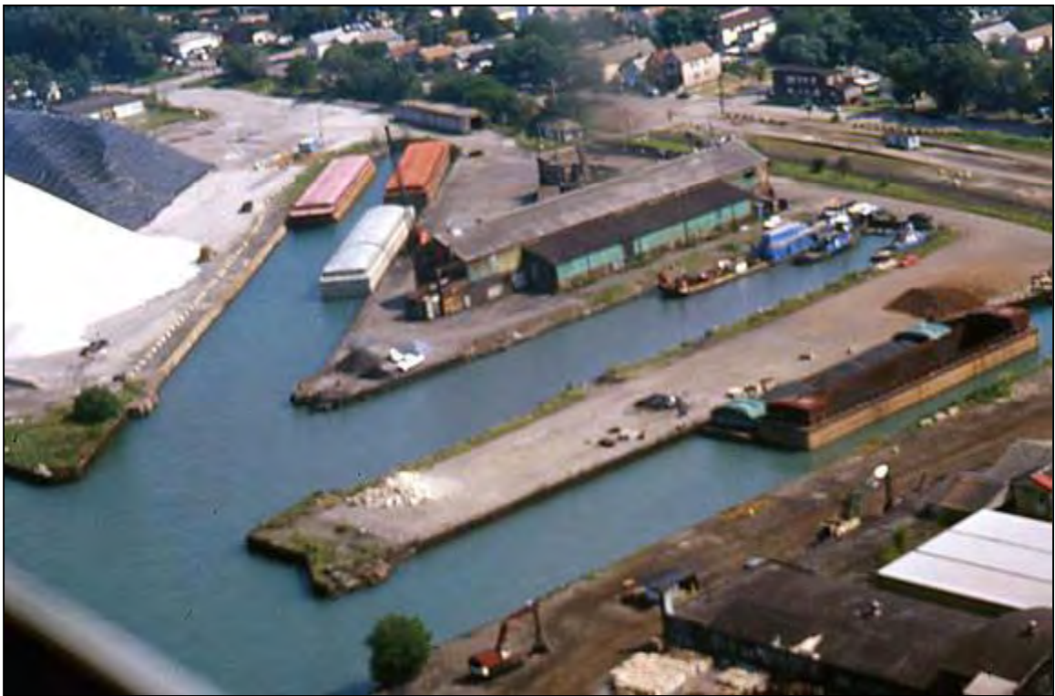
61. Shipyard area, 100th Street aerial view, 08/22/2004
