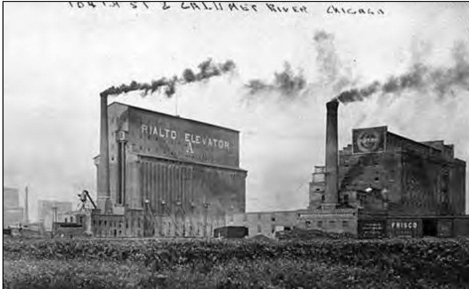
63. Rialto Elevator and Crescent Mills
