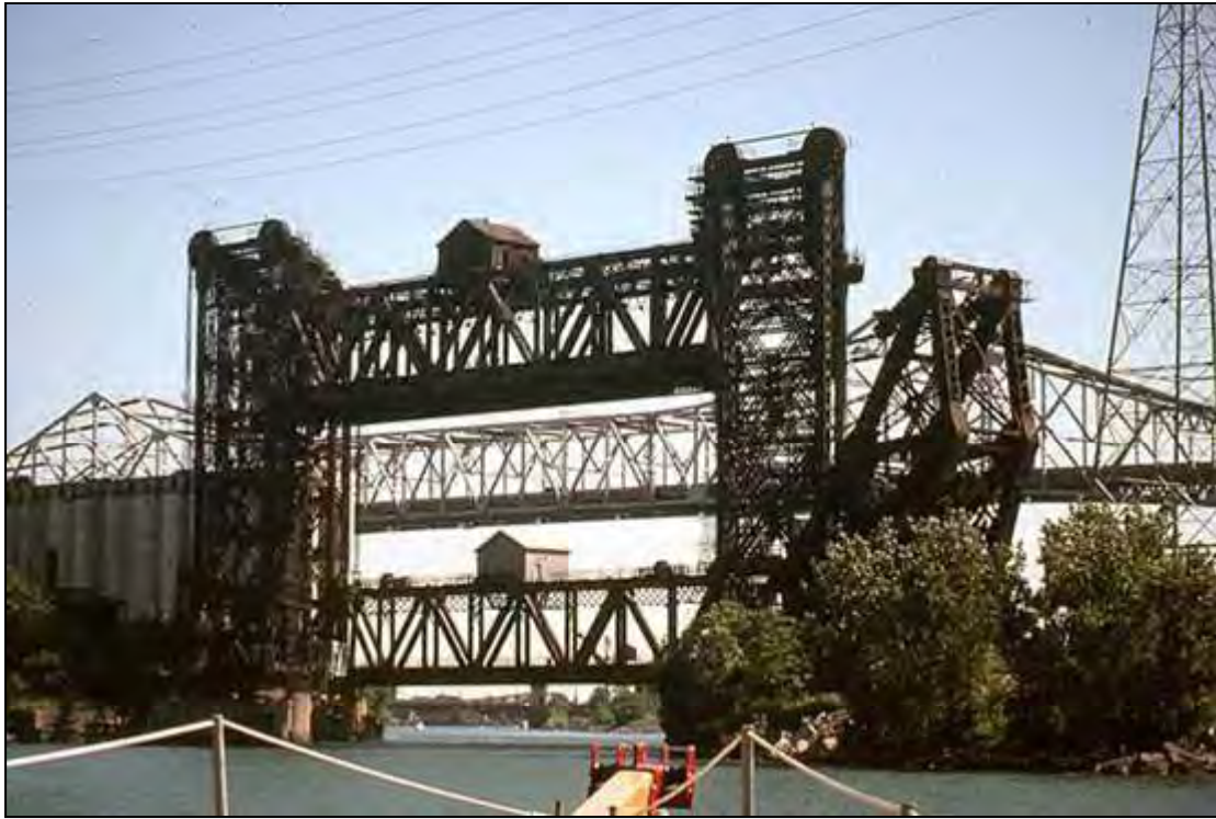
14. RR bridges across Calumet River at 96th Street, July 2000
