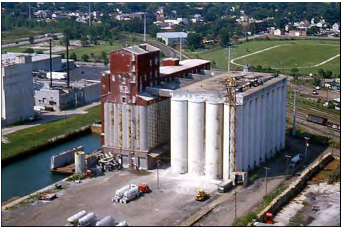
65. General Mills site, aerial view, 8/22/2004
