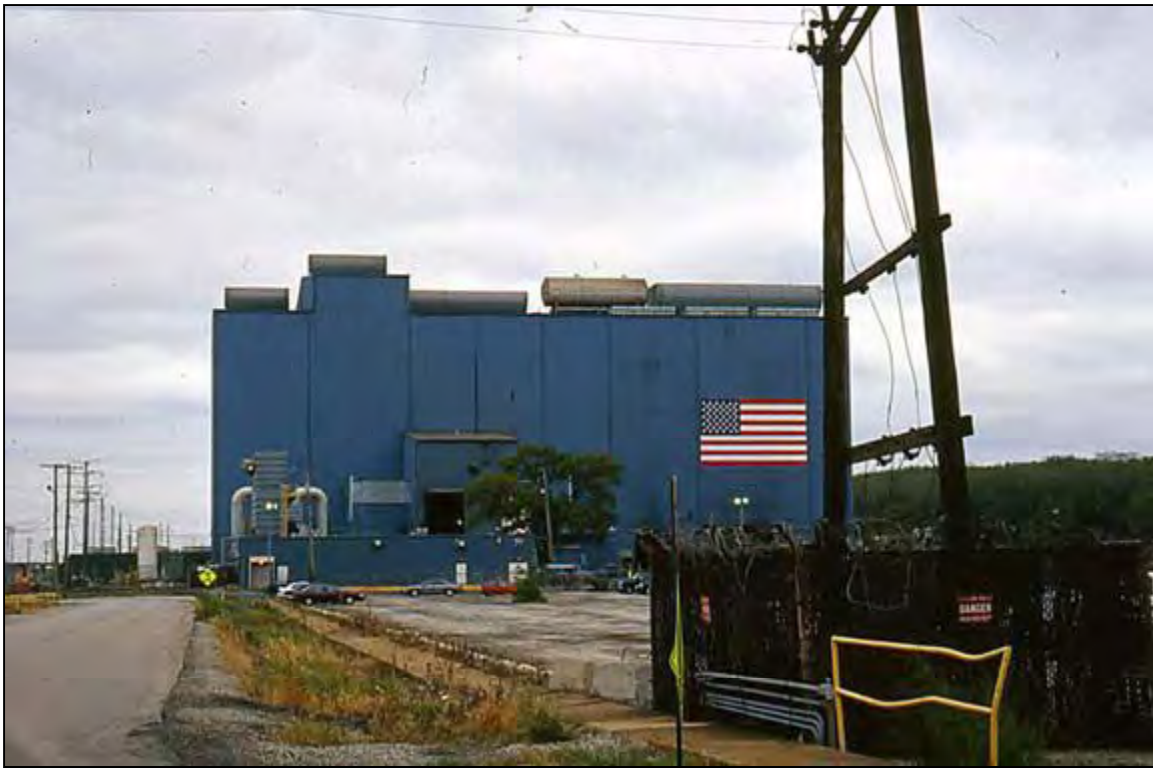
72. Continuous Strip Processor Acme Riverdale, 2005
