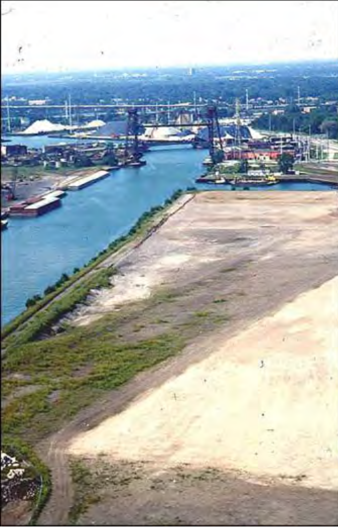
7. Calumet River mouth/EJ&E Railroad bridge from Lake Michigan, 08/22/2004
