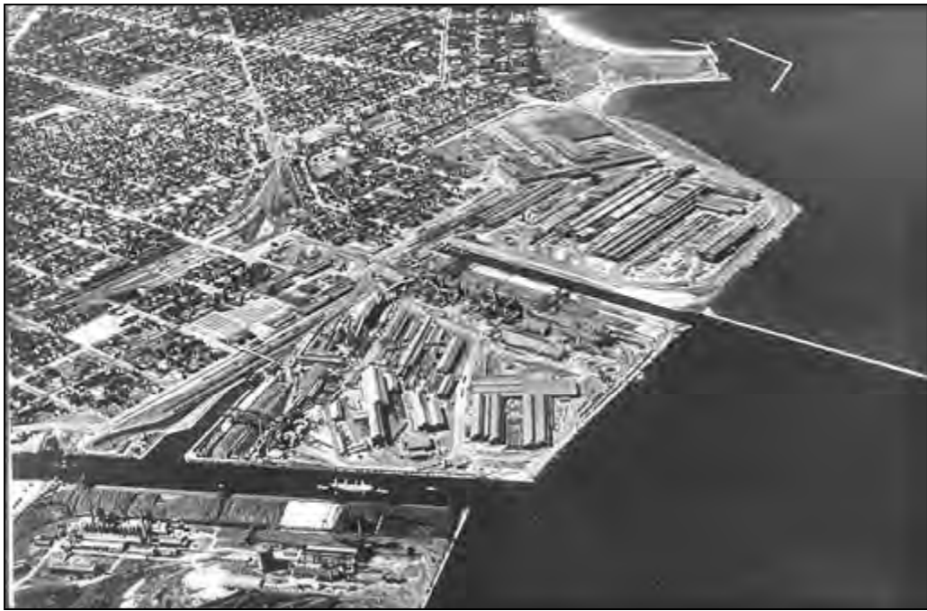
30. USX Aerial – When North Chicago Rolling Mill, the predecessor to US Steel South Works, came to the Southeast Side in 1880 they started with 73 acres of land. Their property had 1500 feet of frontage on the Calumet River and 2500 on Lake Michigan. Slag from the steelmaking process was dumped in a lake front area and this increased the land area for future expansion. This picture shows the furthest extent of the mill which eventually covered over 570 acres.
