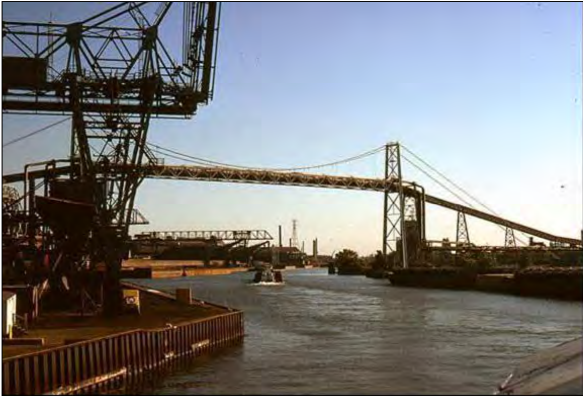
53. Acme conveyor belt over Calumet River at 109th
