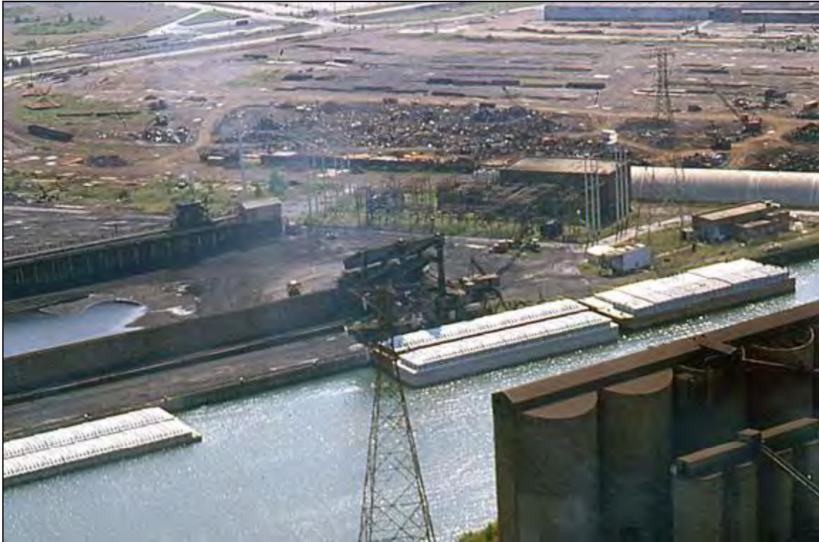
44. Hulett Unloaders, LTV site, aerial view, 8/22/2004
