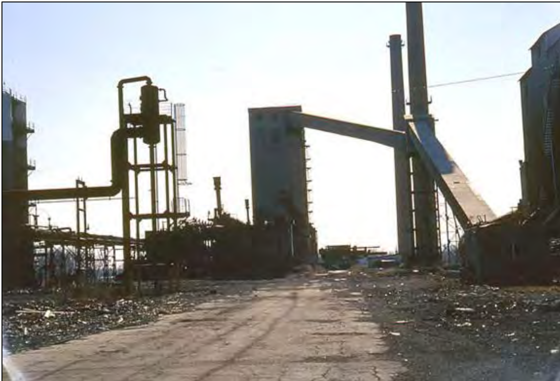
74. Acme Coke view toward coke ovens from north, 2006
