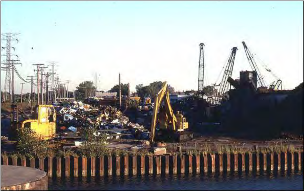
68. Illinois Scrap Processing, view from river, November 1990
