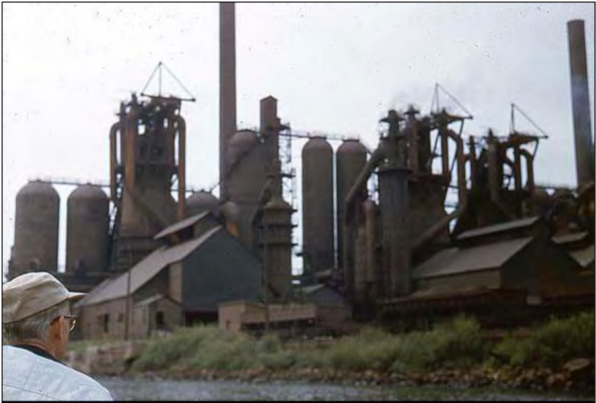
22. Blast Furnaces, August 1, 1954
