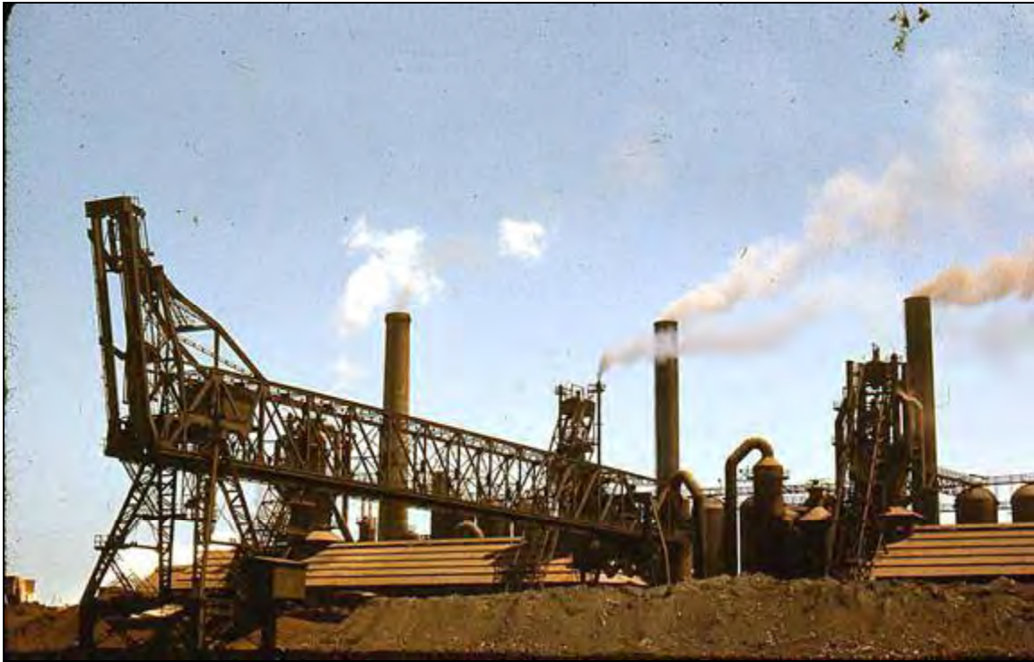
36. Blast Furnaces Youngstown Steel, July 1942
