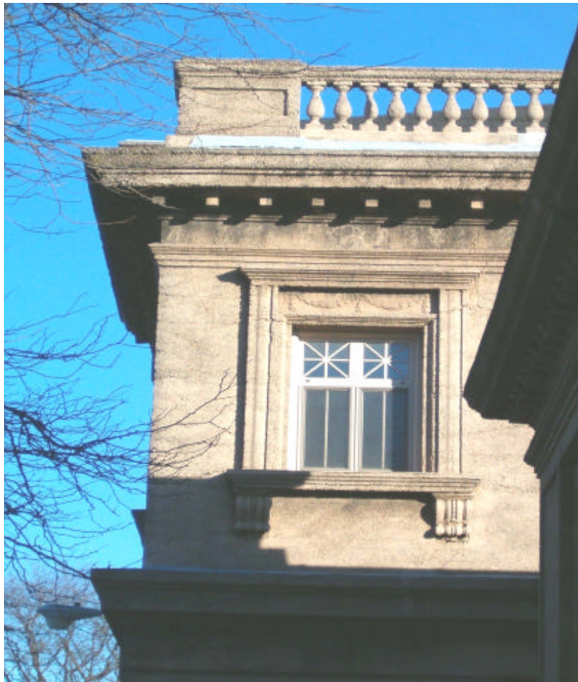
The Calumet Park Fieldhouse incorporates numerous Classical Revival-style elements in its design, including (top) large round-arched windows, and (right) Classical window surrounds, cornice and balustrade.
