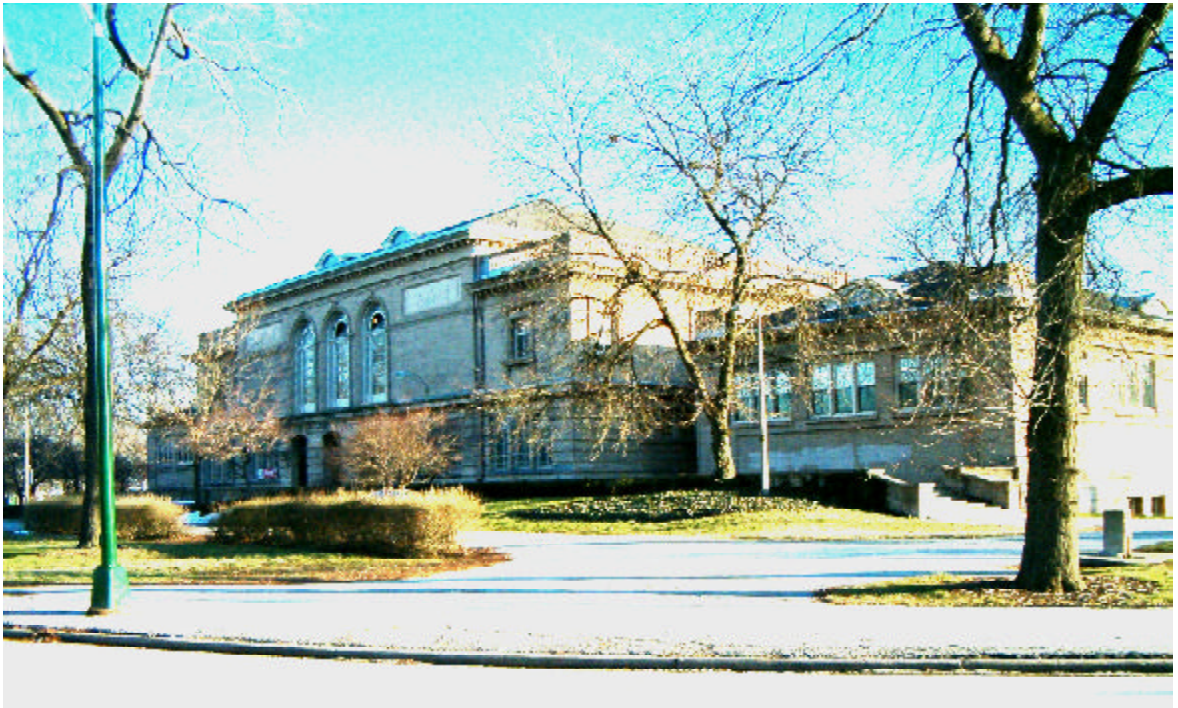
The Calumet Park Fieldhouse has excellent integrity. Top: The fieldhouse shortly after its completion in 1924. Bottom: Calumet Park Fieldhouse in 2006.
