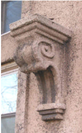
The Calumet Park Fieldhouse's Classical-style details are formed from cast concrete.
