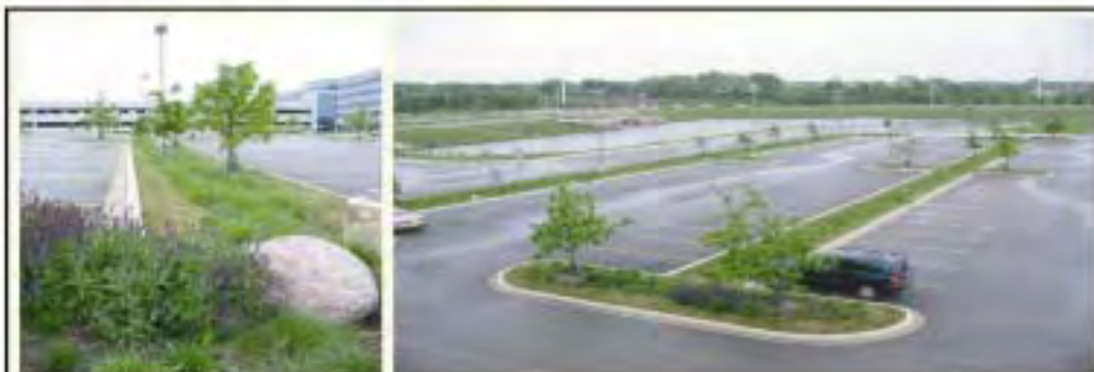
Parking Lot Bioswales
