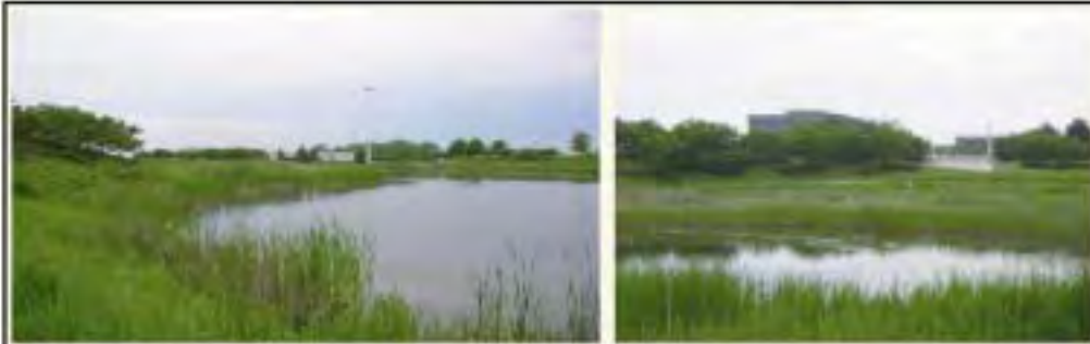
Stormwater Retention - Wetlands
