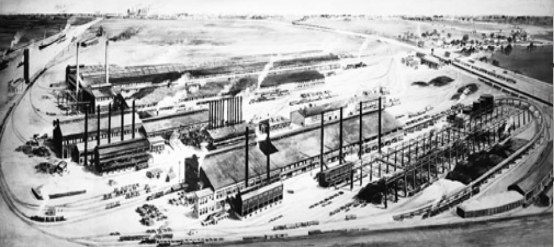
Republic Steel (built 1876) Avenue O & Calumet River
