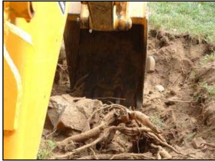
Excavation. Source: http://www.sxc.hu/photo/279748
