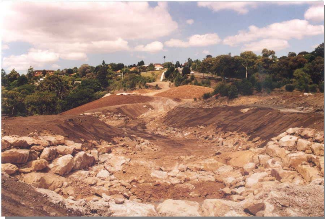
Photo: Flat Rock Gully in 1998 after the council tip site was capped but before revegetation. Photographs obtained from James Smallhorn, Willoughby City Council.
