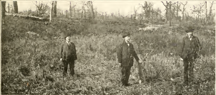
ABOUT TO BREAK GROUND AT GARY
