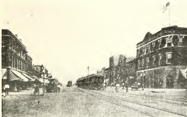
CHICAGO AVENUE EAST OF FORSYTH AVENUE
