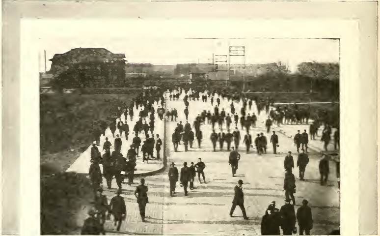
UP BROADWAY TOWARD THE STEEL MILLS
