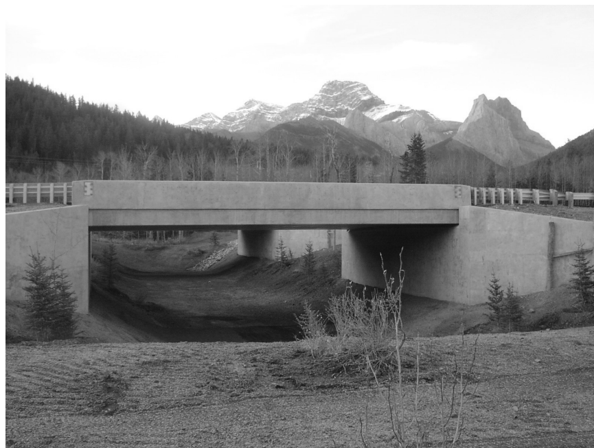
FIGURE 3-4 Wildlife crossings are designed to link critical habitats and provide safe movement of animals across busy roads. Typically they are combined with high fencing and together are proven measures to reduce roadkill and restore movements and regional connectivity. The photograph is of a newly constructed open-span bridge underpass installed on the Trans-Canada Highway near Canmore, Alberta. Source: Photograph by Tony Clevenger, 2005.
