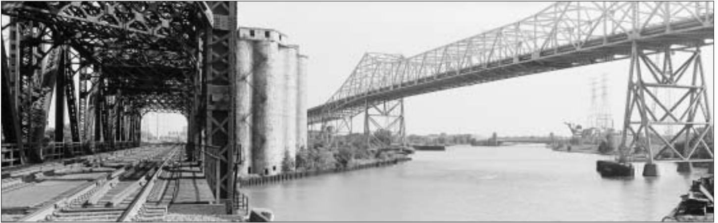
Chicago Skyway and the Waddell and Harrington Lift Bridge over the Calumet River.
