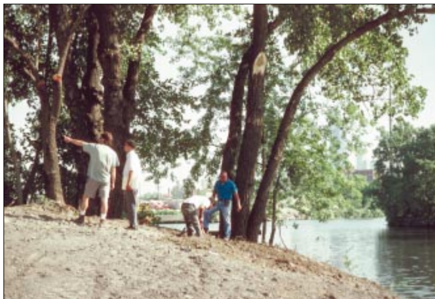
Fellowship House staff worked closely with the Pilsen-based contractor conducting the site grading to facilitate future work to be completed by center youth and local grade school children. Courtesy of National Park Service.
