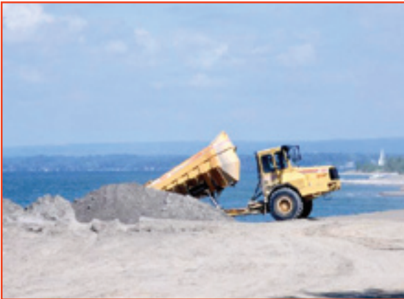
Lake side placement of dredged sand at Presque Isle State Park. Credit: Pennsylvania Dept. of Environmental Protection
