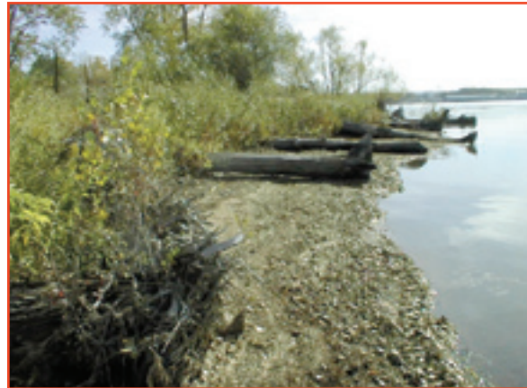
Bay side placement and stabilization of dredged material at Presque Isle State Park. Credit: Pennsylvania Dept. of Environmental Protection.
