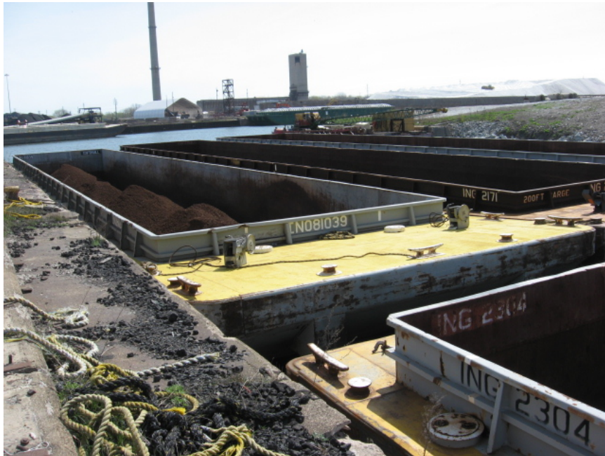
Photo 7. South slip looking east-southeast from the WSW Eastern Coal Storage Area. April 4, 2012.
