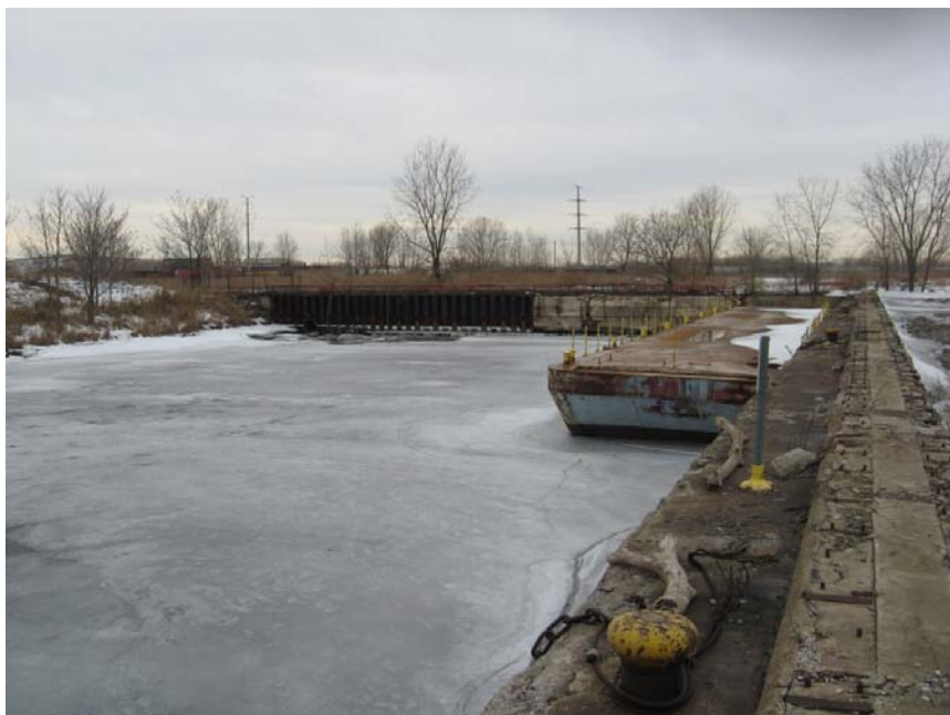
Photo 4. South Slip looking southwest towards sheet pile wall and earthen slope. February 15, 2011.
