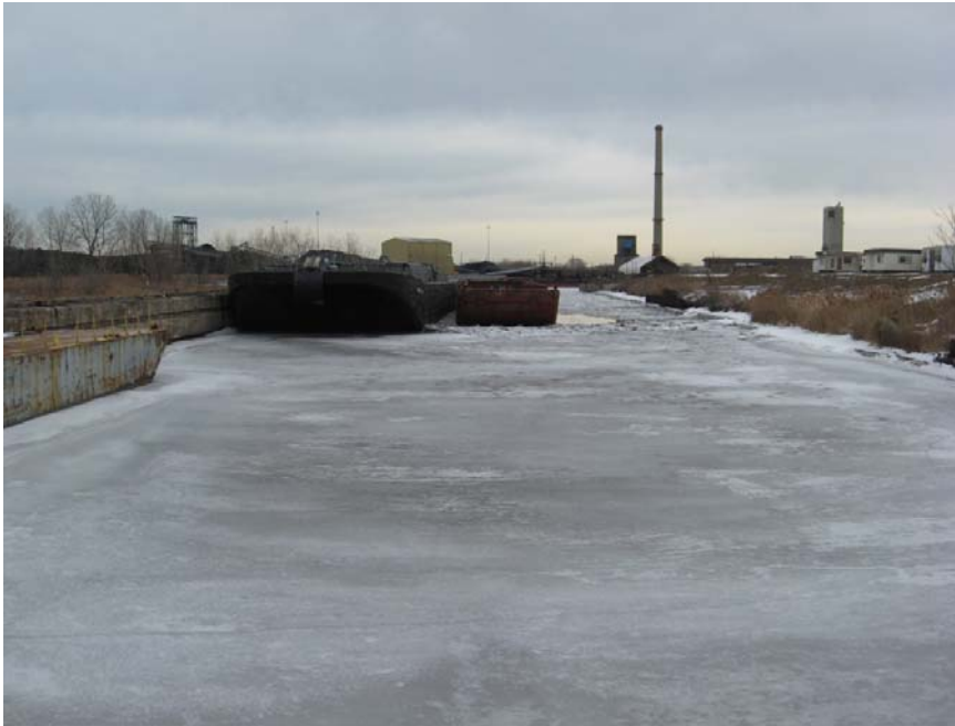
Photo 1. South Slip looking east from western edge of slip with stored barges present. February 15, 2011.
