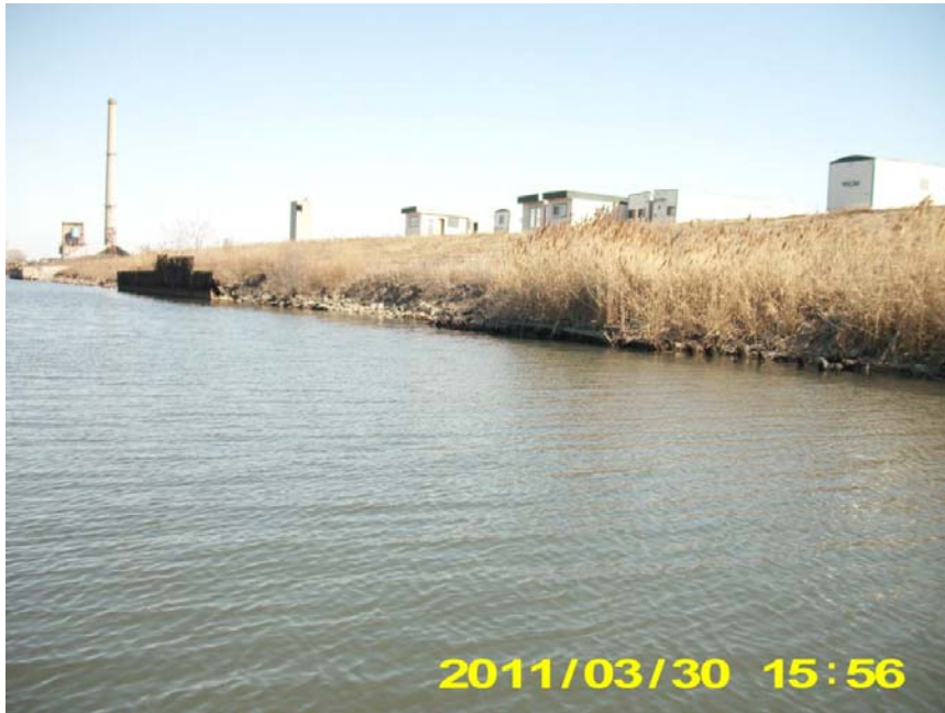
Photo 3. South Slip looking southeast from a barge within the slip towards the earthen slope. March 30, 2011.
