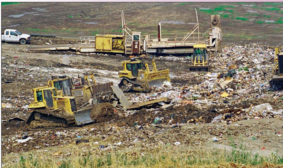
Daily cover operations at an Illinois landfill
