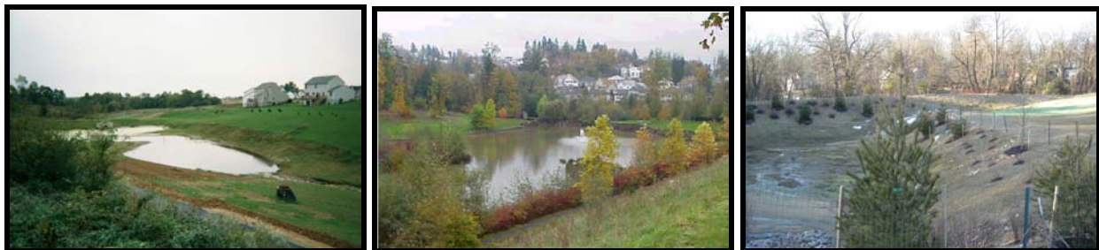
Figure 17. Conventional stormwater pond with no trees (left) and two examples with trees incorporated (center photo source: City of Portland, 2004)
