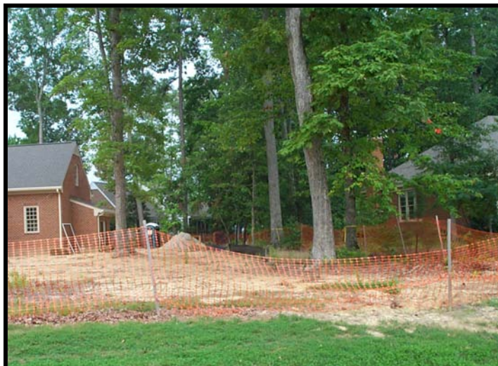
Figure 14. Orange plastic mesh fencing installed to delineate tree protection areas
