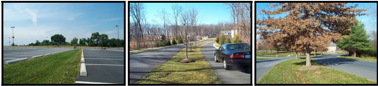
Figure 18. Swale in parking lot with no trees (left), and a swale with trees in a median strip (center and right)
