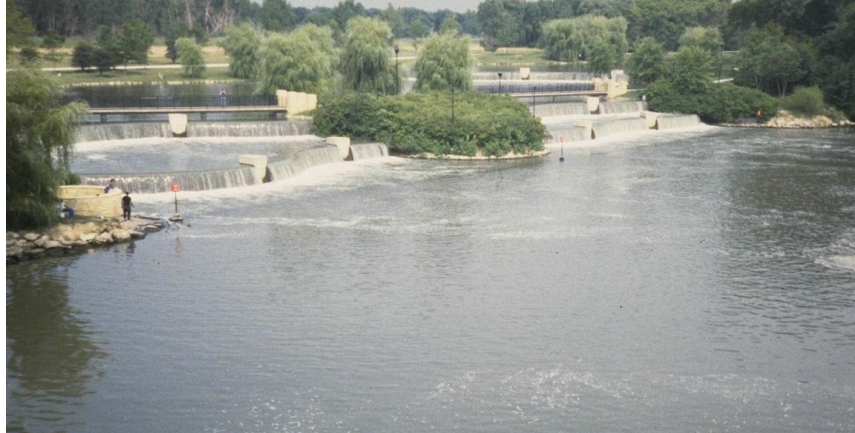
Figure 5. SEPA Station 4 outfall
