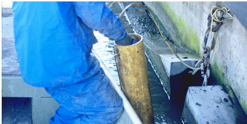
Figure 13. Type II rigging
