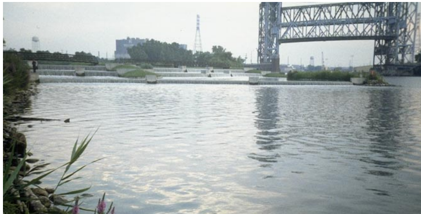
Figure 2. SEPA Station 1 outfall
