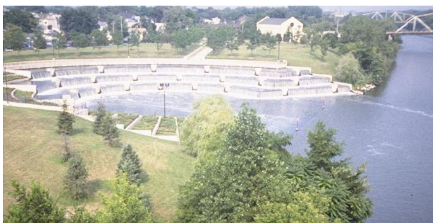
Figure 4. SEPA Station 3 outfall
