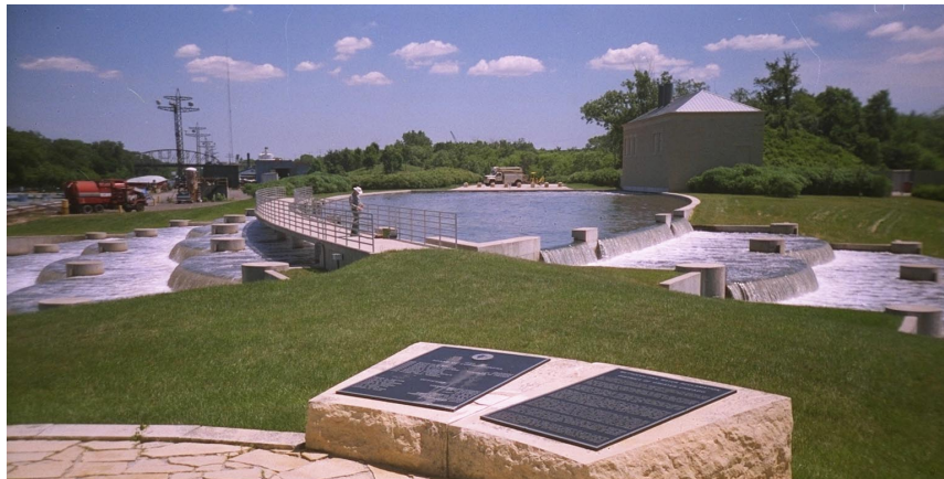
Figure 6. SEPA Station 5 outfalls: Chicago Sanitary and Ship Canal (left) and Cal-Sag Channel (right)
