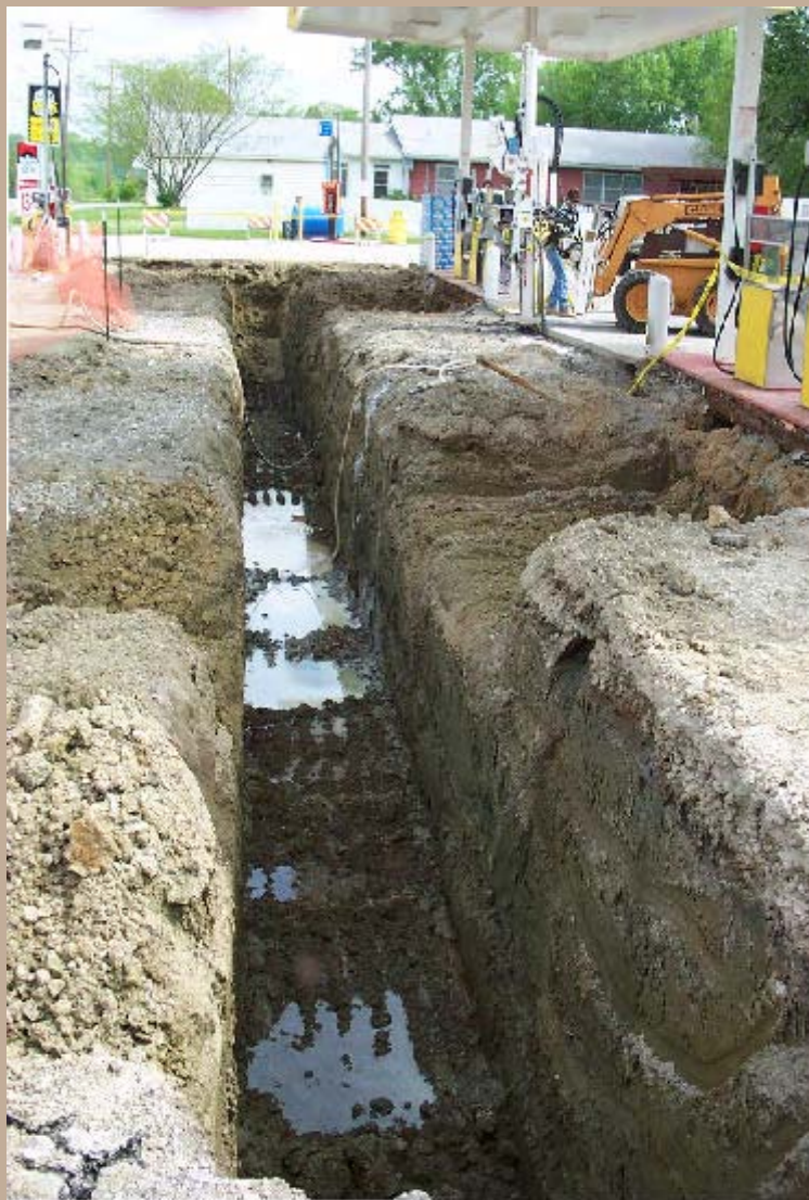
The depth of soil excavation may depend on the groundwater table depth, which may fluctuate due to variable seasonal precipitation.
