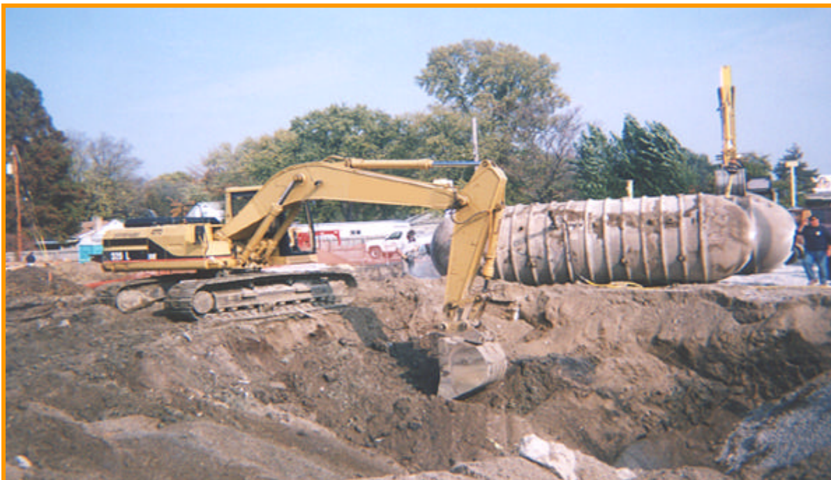
Contractors remove soil in an underground storage tank excavation.
