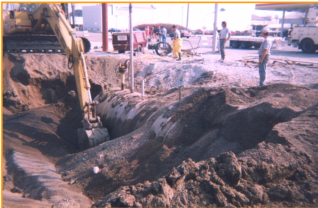
A contractor removes backfill to access the underground storage tank.
