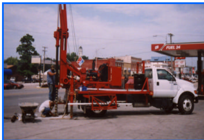
Workers drill a boring to collect soil samples.
