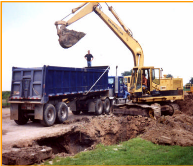
Contractors load excavated soil to be hauled away.
