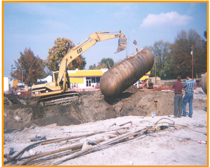
Contractors remove an underground storage tank.
