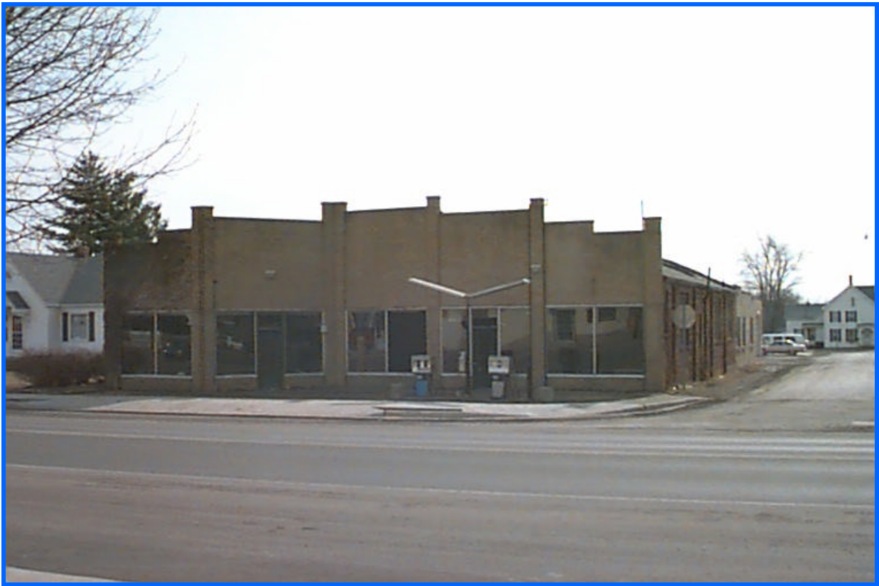
Farmington property slated for redevelopment.
