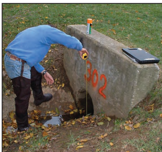
Figure 27: Measuring Outfall Diameter
