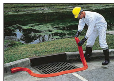
Figure 18: Spill response often involves portable booms and pumps
