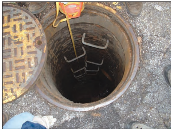
Figure 56: Techniques to sample from the storm drain
