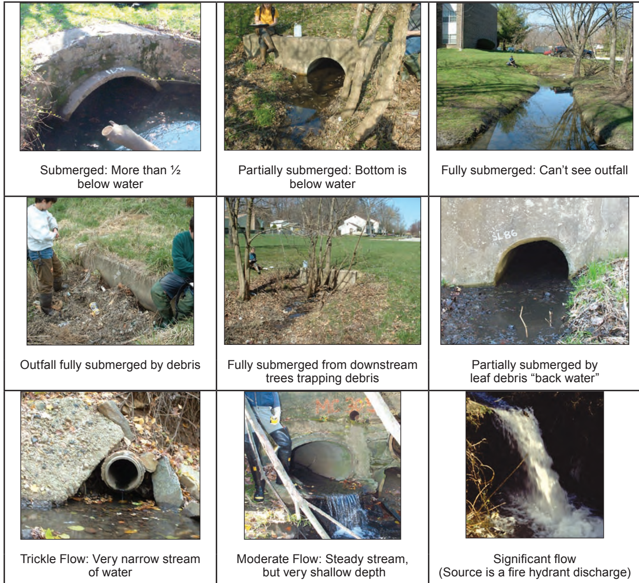
Figure 28: Characterizing Submersion and Flow
