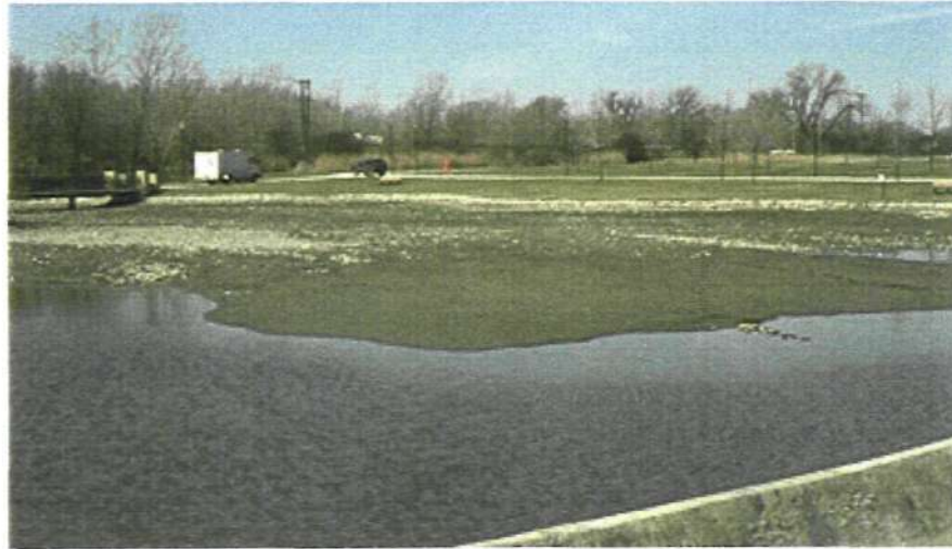
Figure 32. Sediment deposition in SEPA Station 4 distribution pool, spring 1996
