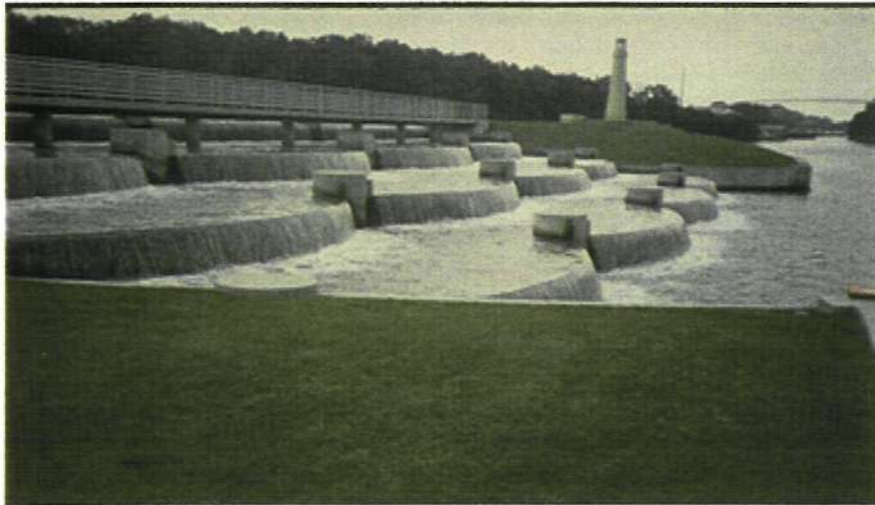
Figure 12. SEPA Station 5 discharge weir to Chicago Sanitary and Ship Canal, summer 1996
