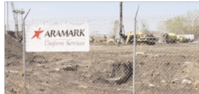
Construction has begun at the new Aramark manufacturing facility
