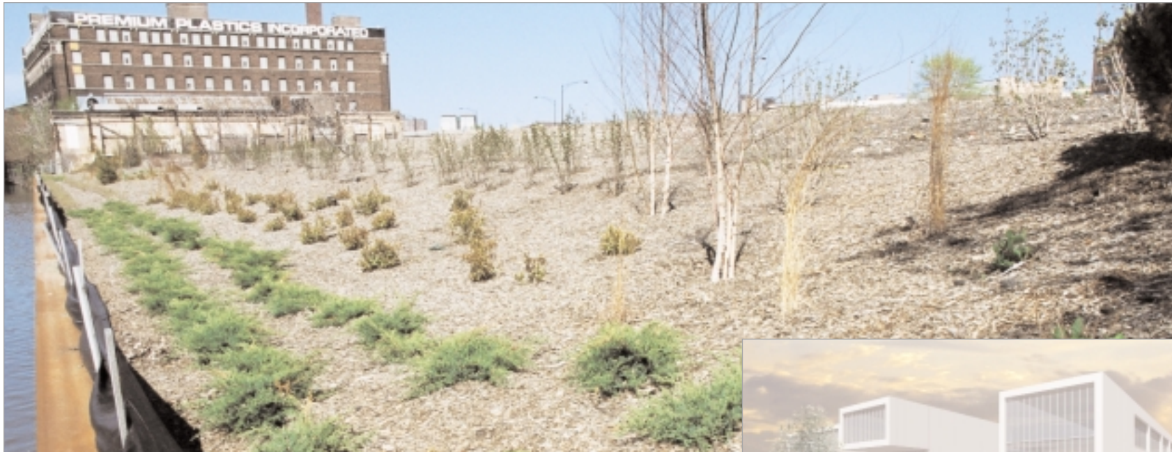
Work has begun at the International Union of Operating Engineers' site
