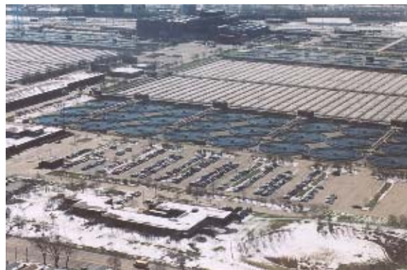
Stickney WRP is the largest WWTP in the world.
