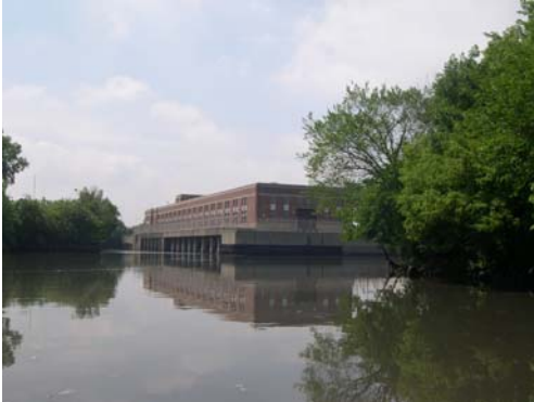
Racine Avenue Pumping Station provides flow for the South Branch when it discharges.
