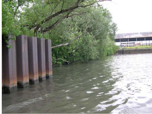
Mixture of sheet pile bank and overhanging vegetation in the SBCR
