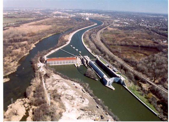
Lockport Powerhouse and Lock is the main outlet control for CAWS.
