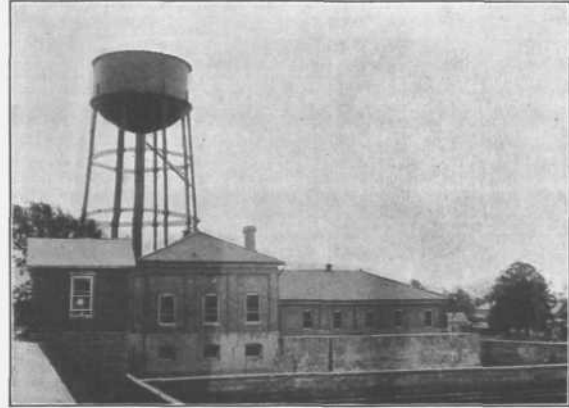
Figure 6.—Filter house and elevator tank, Eock Island.
