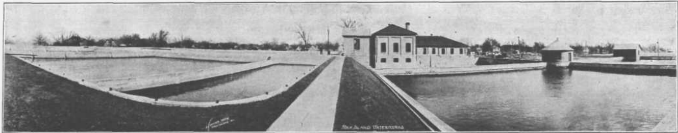
Figure 7.—Filtration plant, Rock Island.
