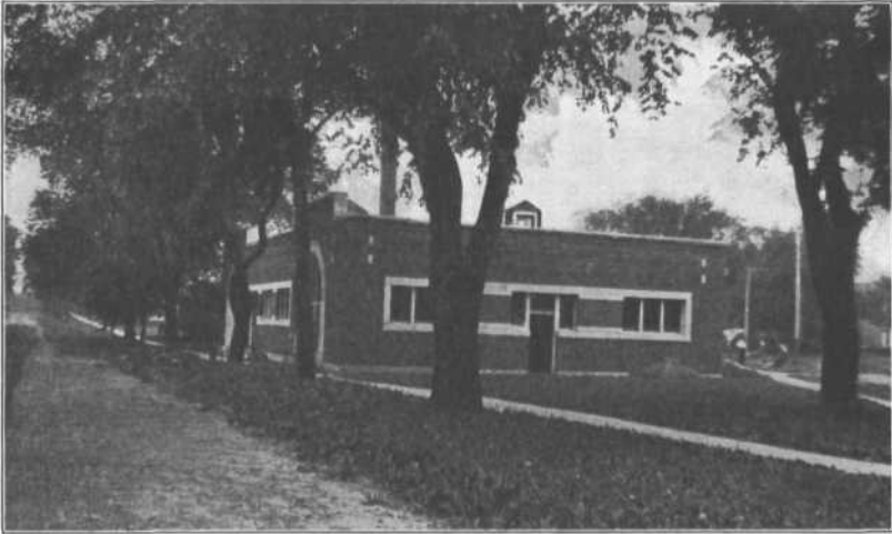
Figure 1.—Waterworks pumping station, Arlington Heights.
