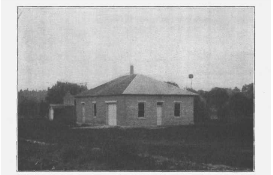
Figure 2.—Well house and pumping station, Carpentersville.
