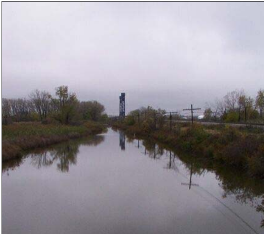
Figure 24: Structure #17 - Looking South From 122 nd Street.
