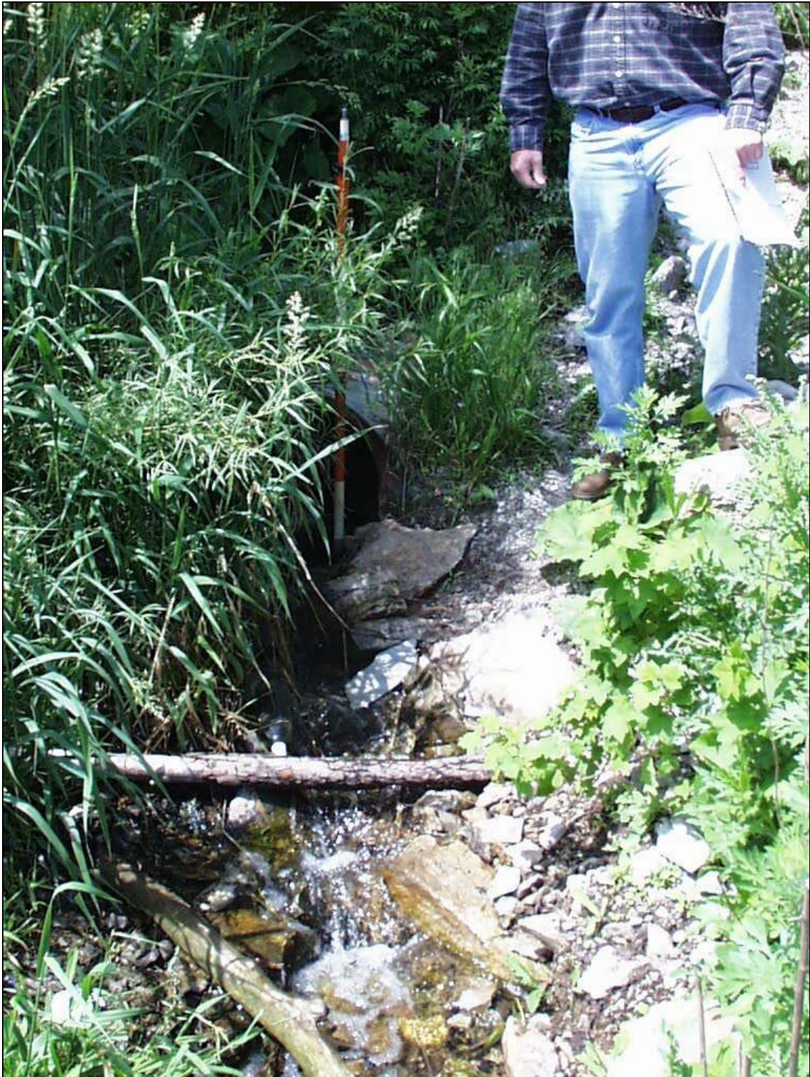
Figure 5: Structure #1 - Outlet Pipe and Channel.
