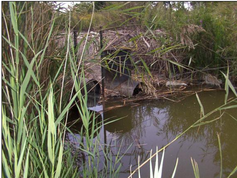
Figure 20: Structure #15 - Looking South.
