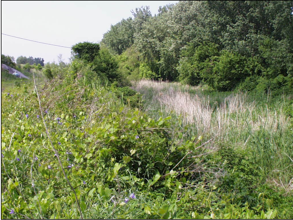
Figure 23: Structure #17 - Downstream End Looking North.
