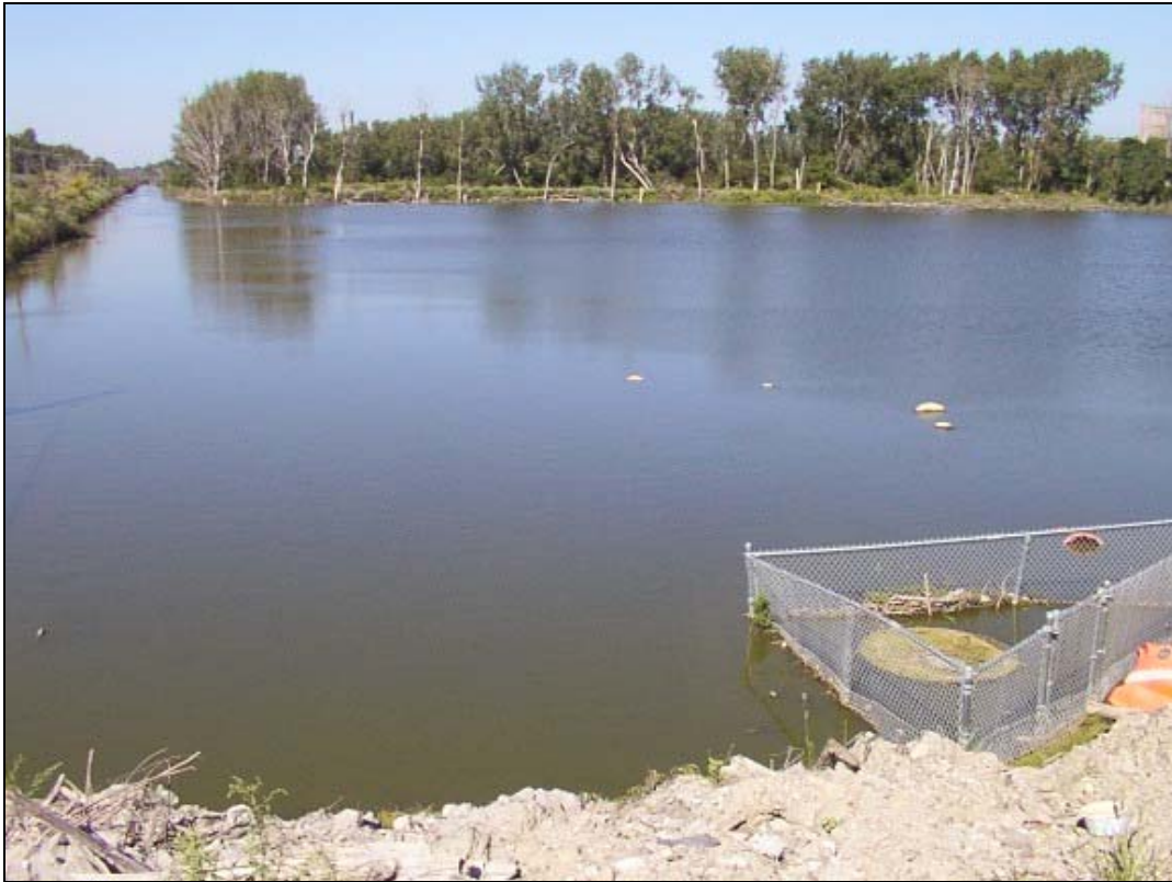
Figure 10: Structure #3 - Looking North.
