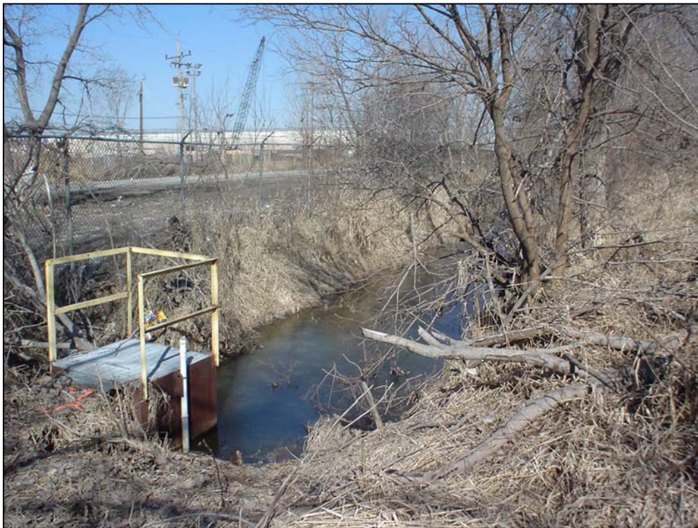
Figure 3: Structure #1 - Approach Channel.
