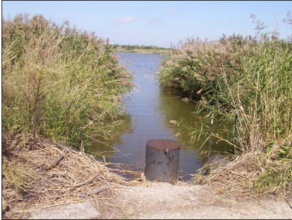
Figure 19: Structure #15 - Looking North.
