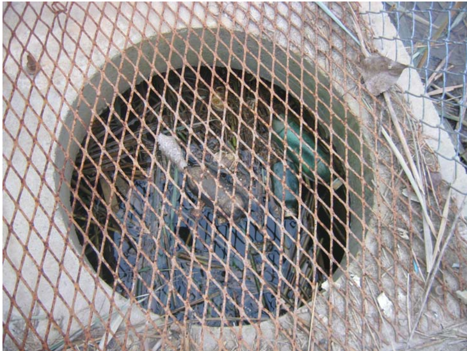
Figure 14: Structure #5 – Looking Inside Structure.
