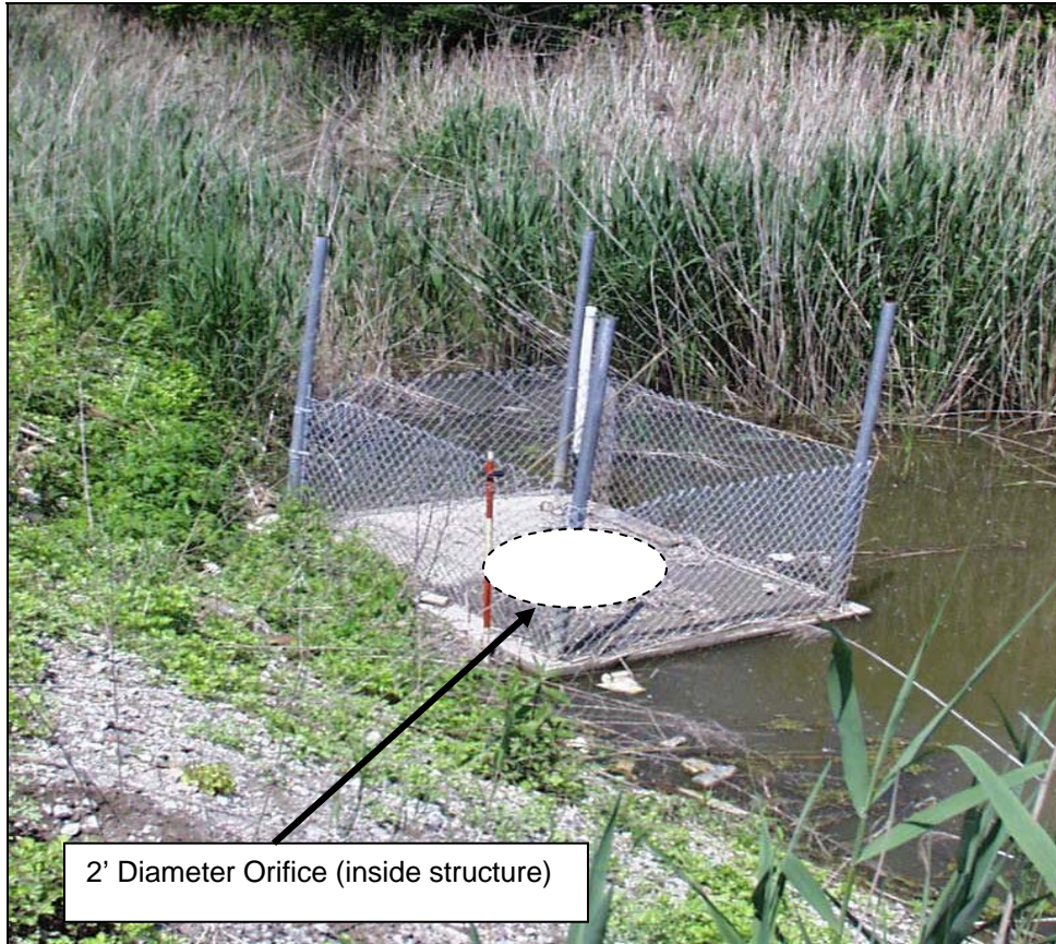
Figure 13: Structure # 5 – Looking North.
