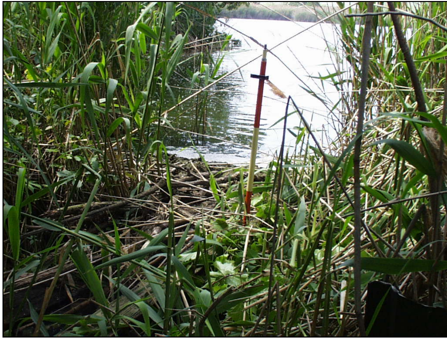
Figure 7: Structure #2 – Weir Constructed of Grass and Debris.
