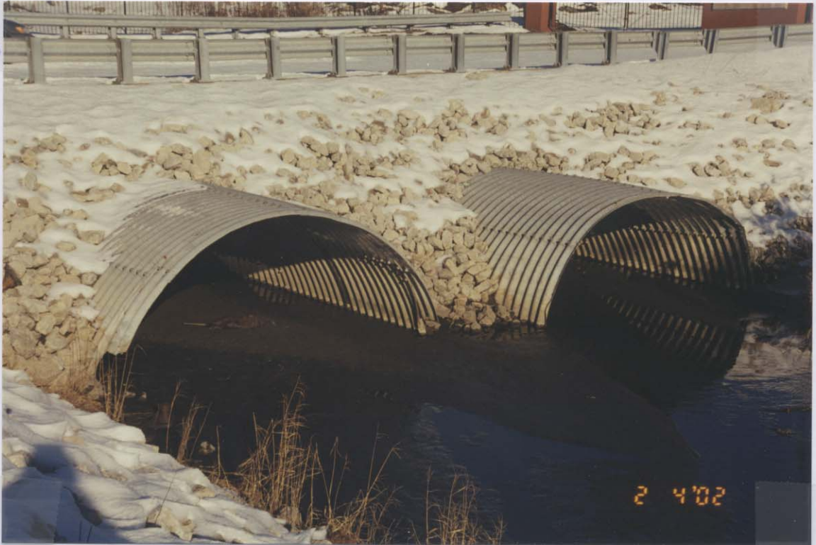
PULLMAN CREEK CULVERTS
