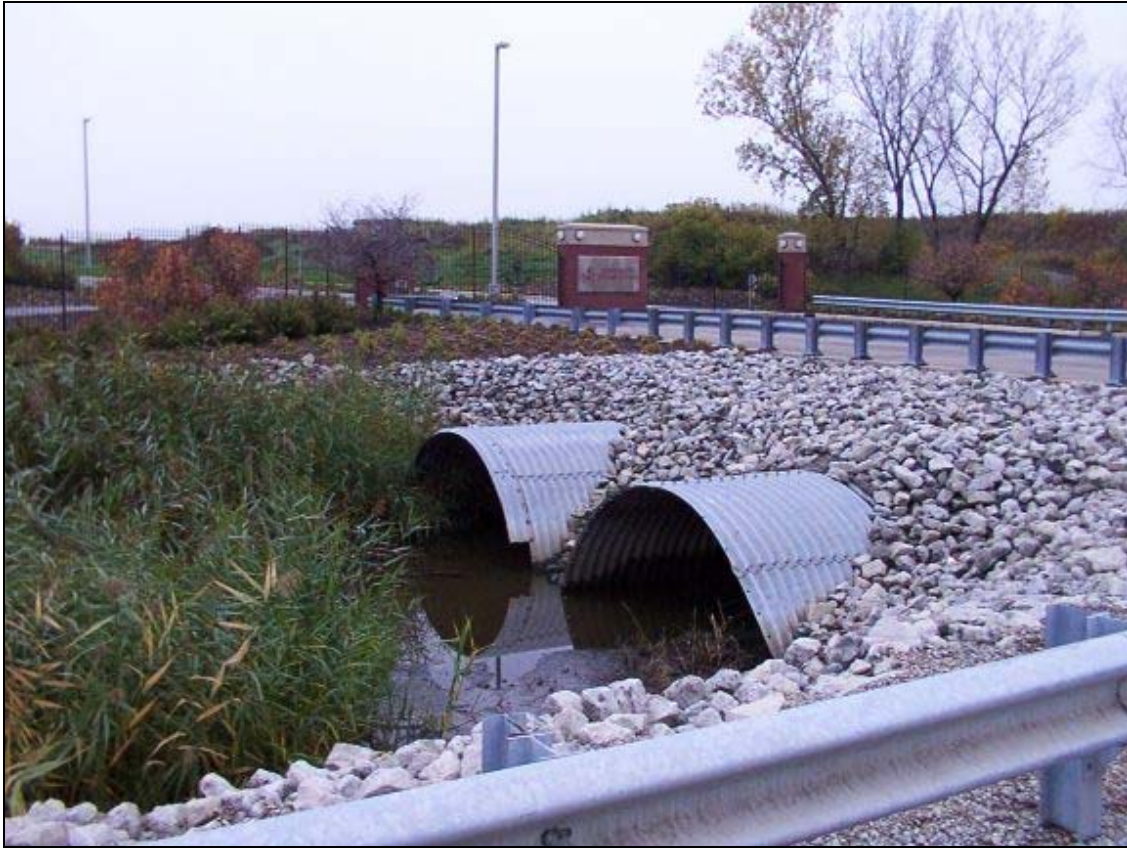
Figure 3: Golf Course Access Driveway with Arch Culverts.
