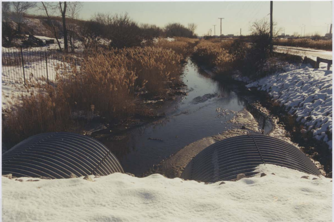
PULLMAN CREEK LOOKING SOUTH (BRIDGE #2)
