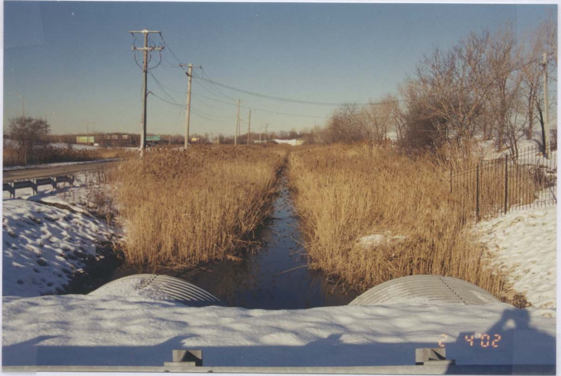
PULLMAN CREEK LOOKING NORTH (BRIDGE #2)
