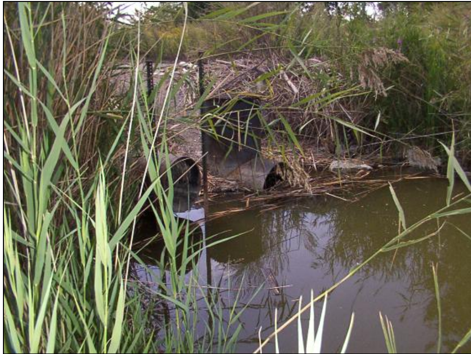
Figure 32: Structure #15 - Looking South.
