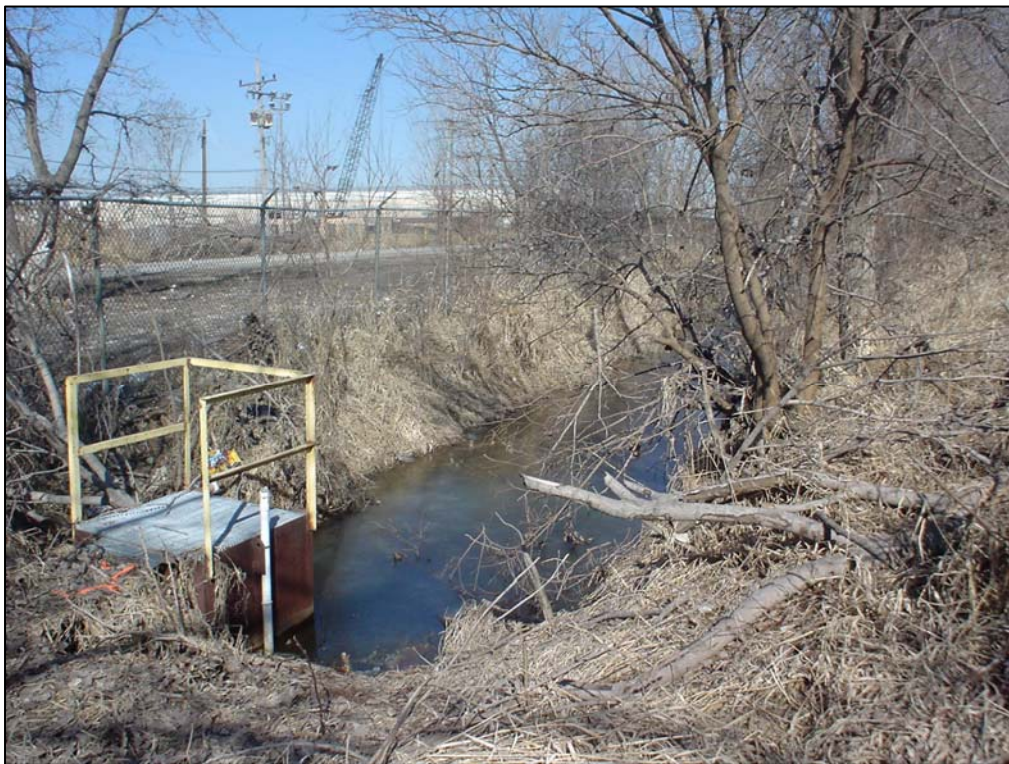
Figure 5: Structure #1 - Approach Channel.
