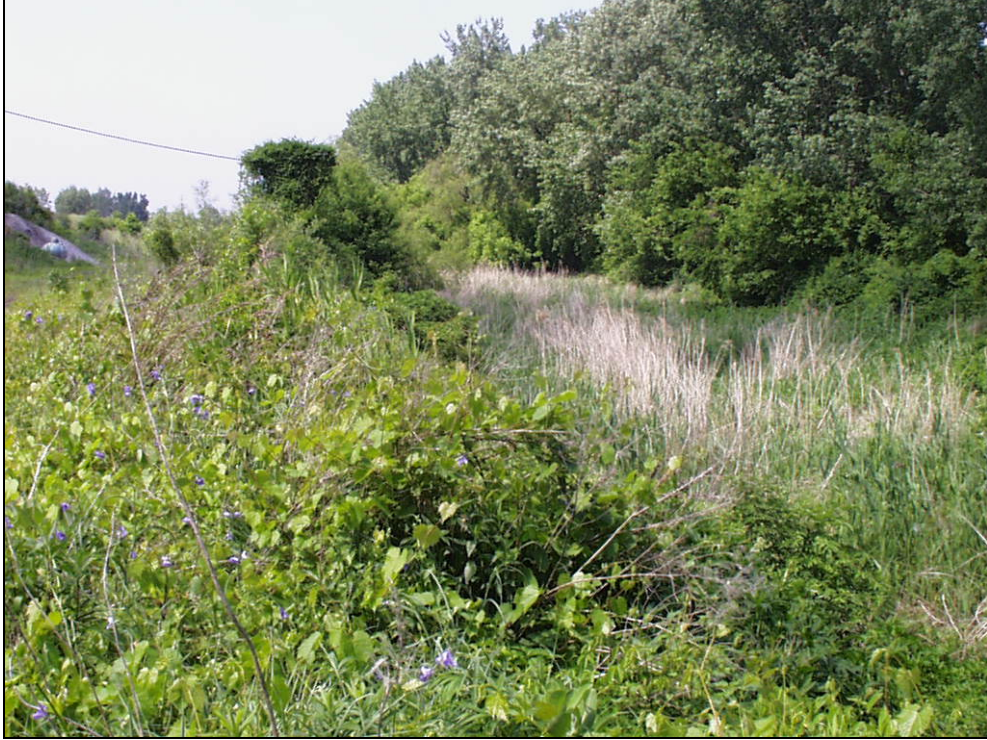
Figure 36: Structure #17 - Downstream End Looking North.
