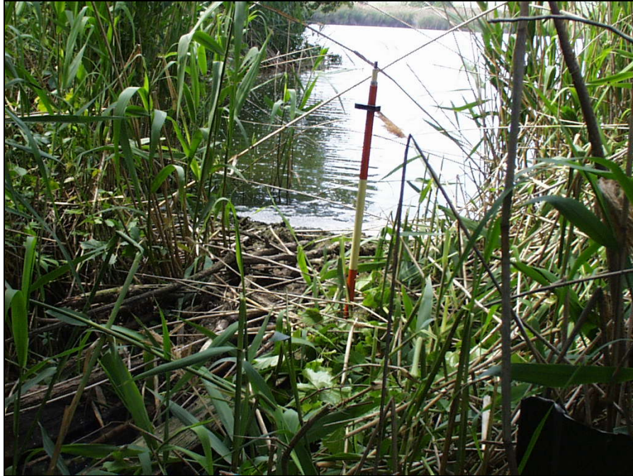
Figure 10: Structure #2 – Weir Constructed of Grass and Debris.
