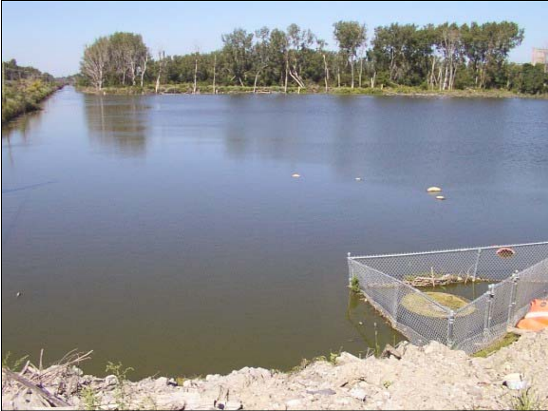
Figure 14 – Structure #3 Looking North.
