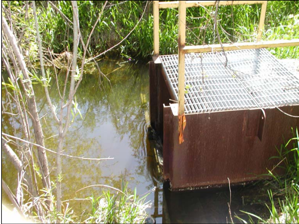
Figure 4: Structure #1 - Looking East.
