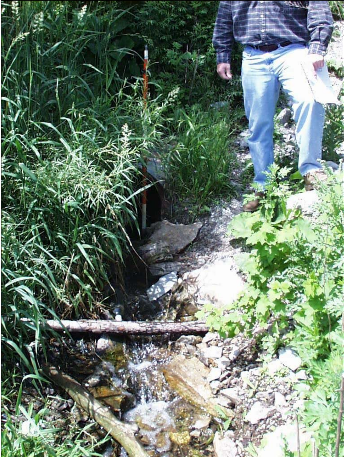
Figure 7: Structure #1 - Outlet Pipe and Channel.
