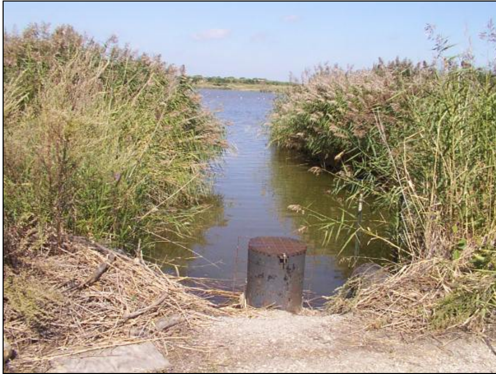
Figure 31: Structure #15 - Looking North.
