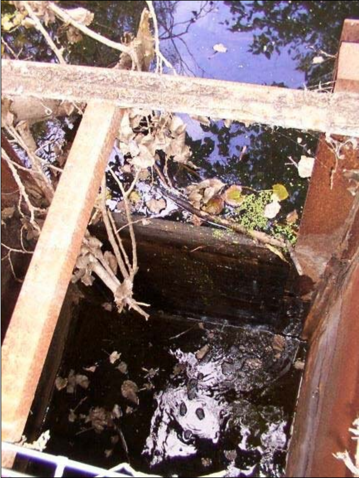
Figure 6: Structure #1 - Inside View.
