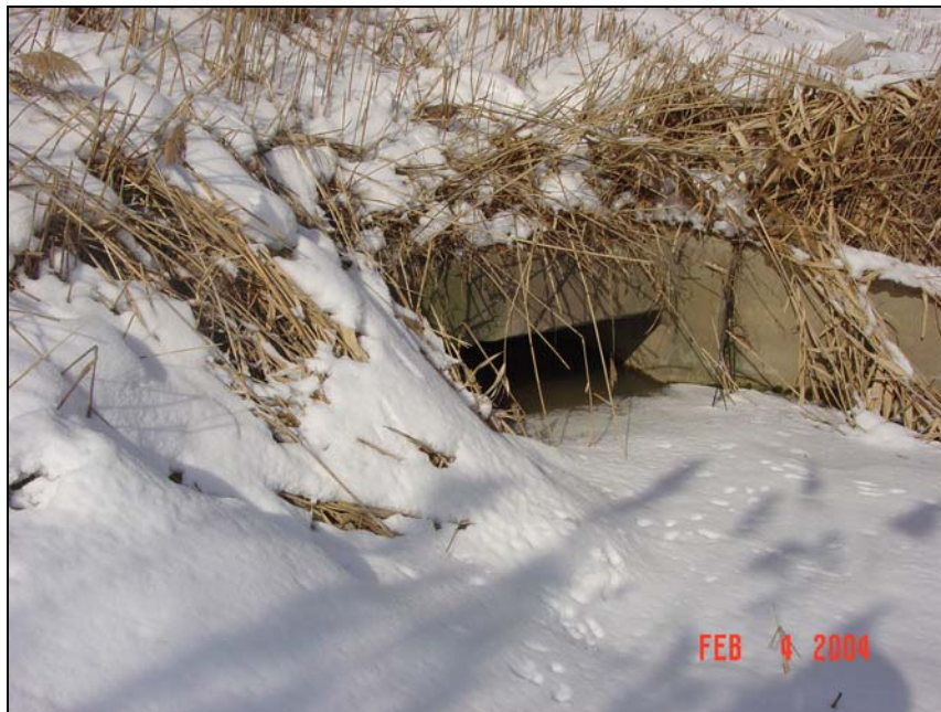
Figure 26: Structure #11 – Box Culvert Under Doty Avenue at 110 th Street.
