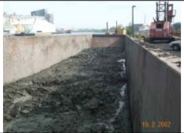
Fig. 4. In Chicago on October 2 the barge contains little free water. Four truckloads were removed that day.
