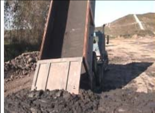
Fig. 17. The dredged material generally flowed smoothly from the trucks.
