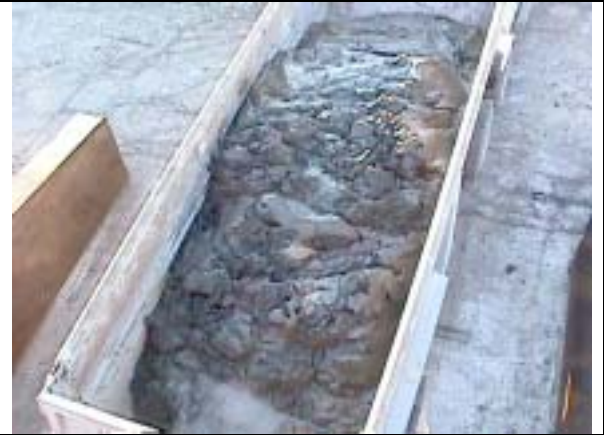
Fig. 10. The sediment maintained its consistency and piled inside the trucks.
