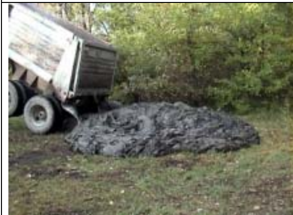
Fig. 11. Material placed at the William Powers Conservation Area made distinct piles about 30 inches high when dumped in one spot.
