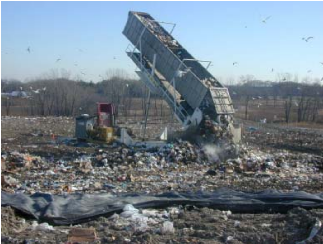
Tipper in active working face at Onyx Zion Landfill Site 2, which ranks sixth in Illinois in terms of waste disposed, and eighth in terms of capacity
